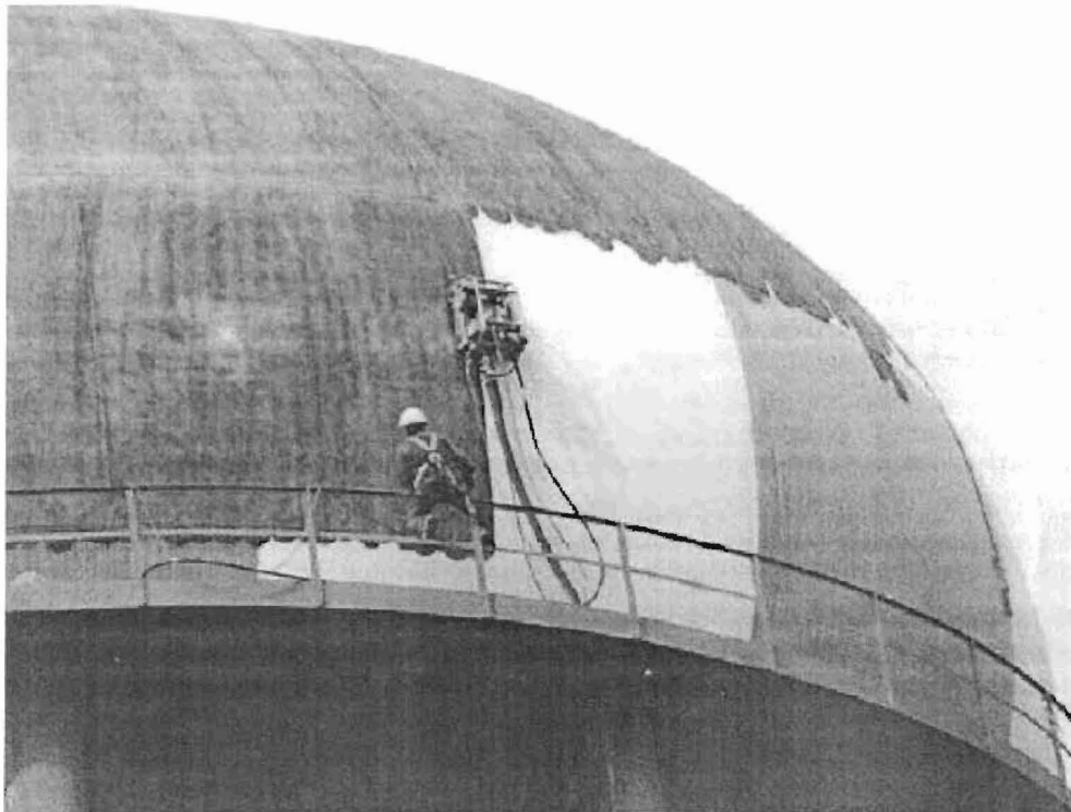
Figure 3: A water-jet surface preparation machine
