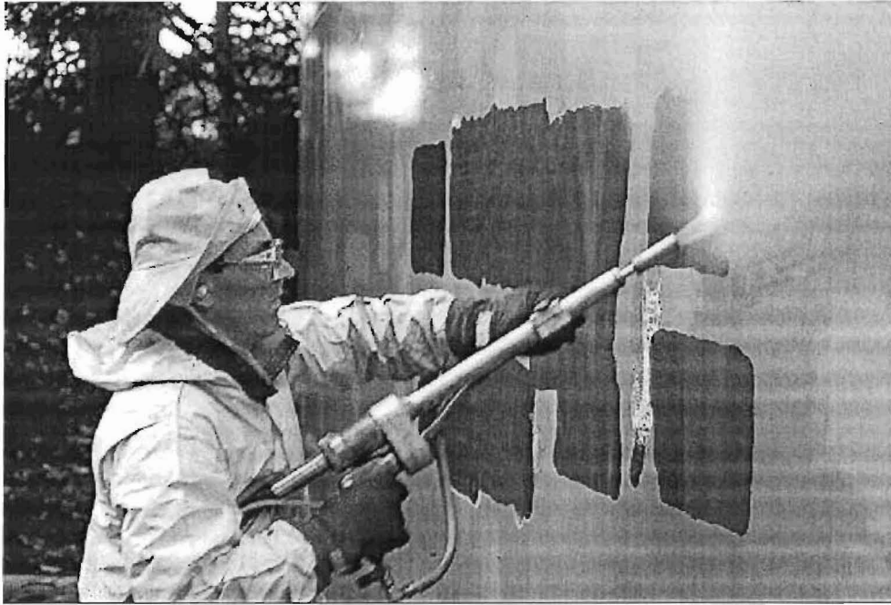
Figure 2: A water-jet cleaning “wand”
