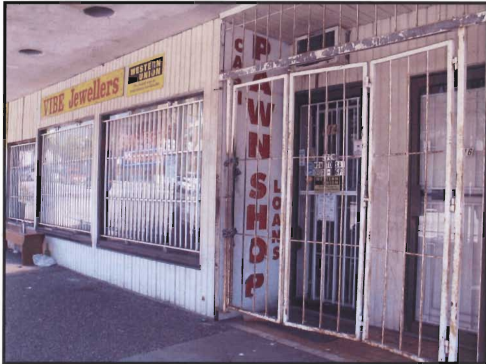
Unattractive security bars across a shop's windows and door on Columbia Street send a message that the area is not safe (Photo: J. Natland)
