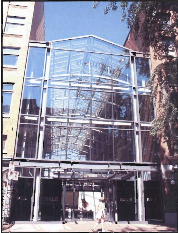
Exterior walls of heritage buildings in Gastown, Vancouver serve as interior walls of newer building (Photo: J. Natland)
