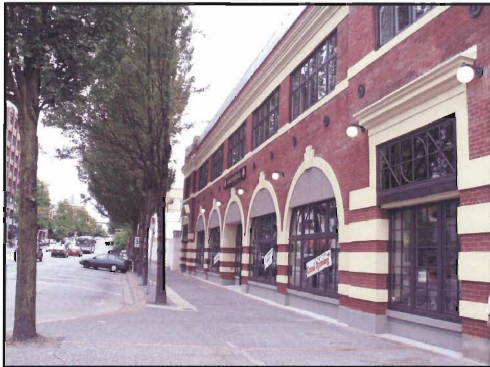
Arched windows along front façade of 774 Columbia Street (Photo: J. Natland)
