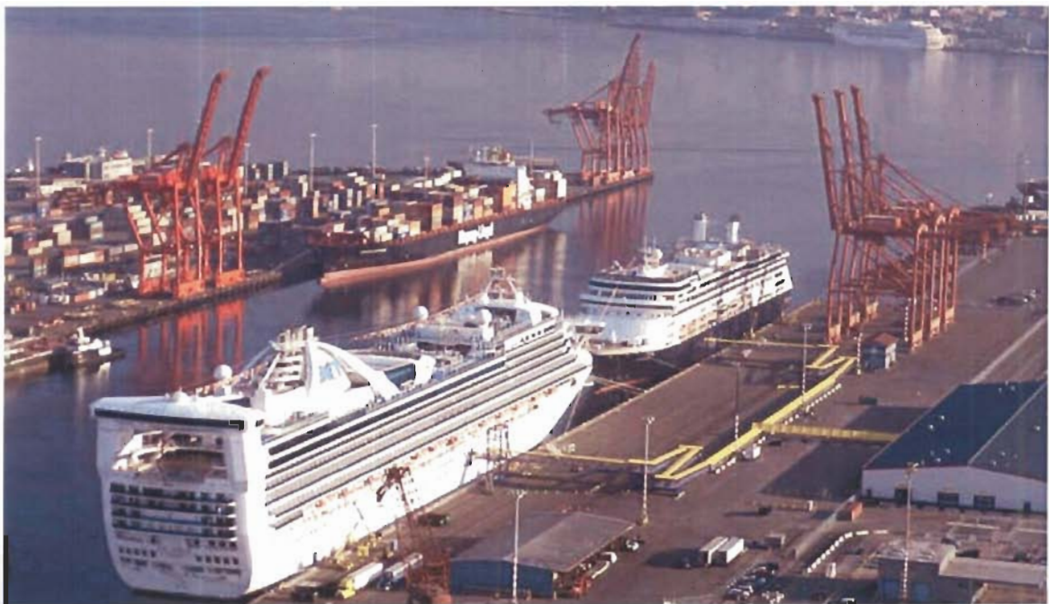
Figure 2-11: Port of Seattle's Terminal 30 Cruise Ship Terminal
