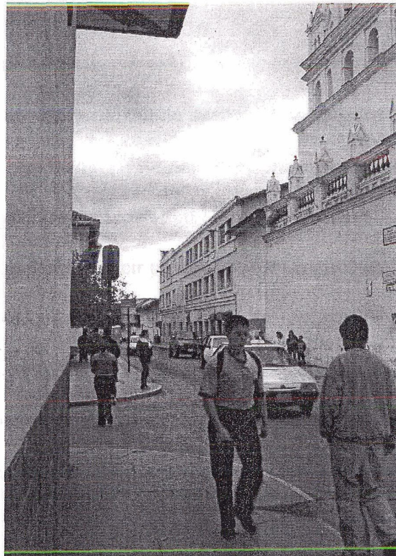
Figure 5. North Wall of Convent: the espadaña of the church (right) was completed in the late 19 th century. The three storey building (center) built in 1965 now contains the offices of the convent, the torno , porteria , and locutorio .
