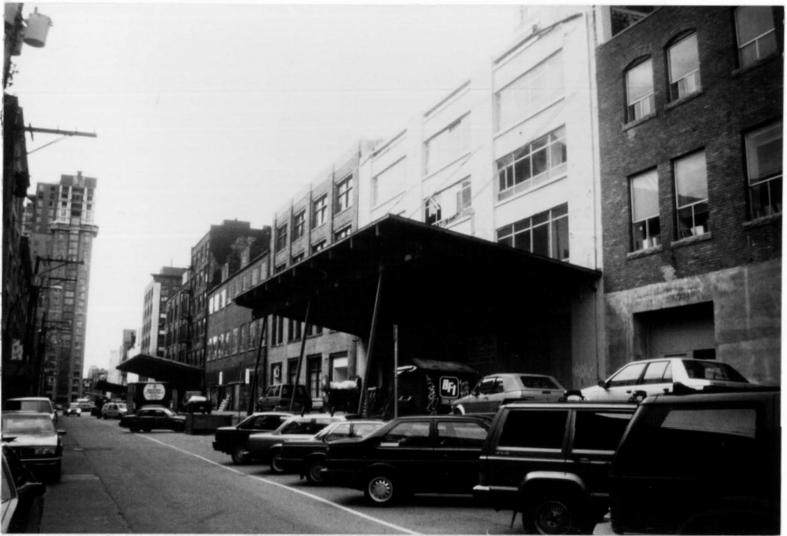
Figure 3.1 Yaletown Warehouses and Loading Docks
