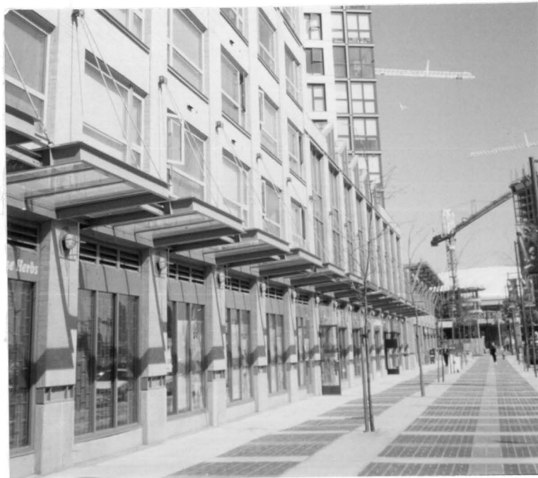
Figure 3.4 Overhanging Canopy and Brick Facade of Concord Pacific Building
