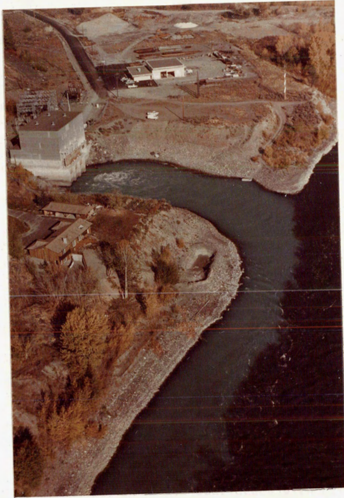
PLATE 1. Seton Lake water discharged into the Fraser River at Seton powerhouse.
