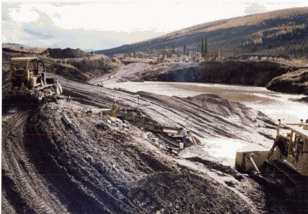
Typical settling pond. A large portion of the clay/silt fraction is not removed and passes through the settling pond and downstream.
