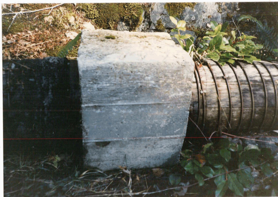
Plate 5: PENSTOCK THRUSTBLOCK. (Koksilah Power Company, March 1986.)
