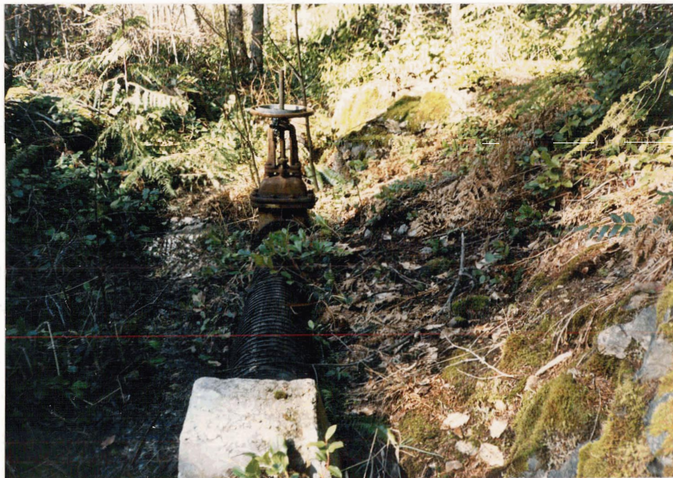
Plate 3: SHUTOFF VALVE NEAR INTAKE. (Koksilah Power Company, March 1986.)
