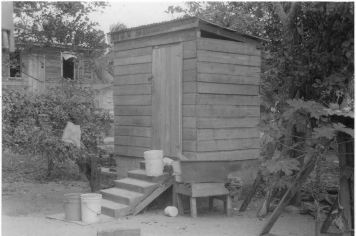
Figure 5.1: A completed and in-use composting toilet
