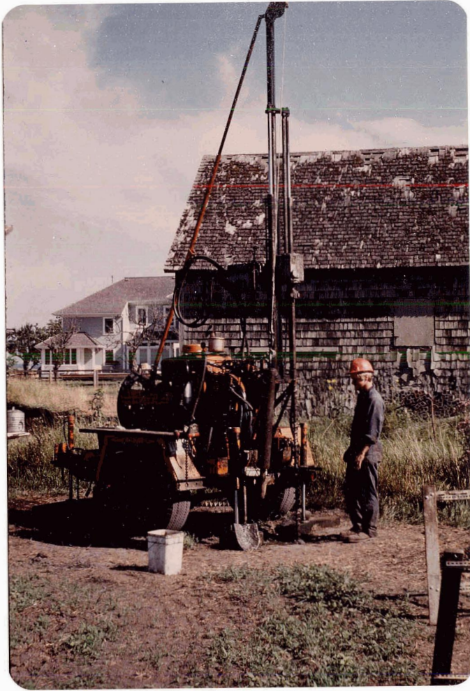
Figure 6.1 Concore C-68 drill rig
