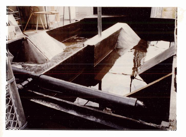
pool a 75 x 95 cm (depth x length) window of 10 mm tempered float glass was installed so that both predators and prey could be observed from an underwater vantage point. A small observation hut was constructed around the window so that extraneous light would not leak into the channel.
