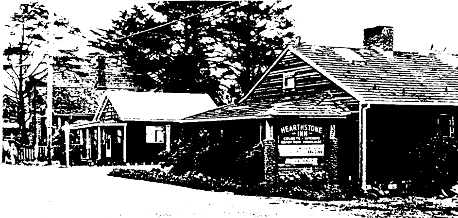
Figure 55: The Hearthstone Inn and a close residential relative, on Hemlock Street in mid town Cannon Beach. (Map 12) The 'Oregon barn' style house, with overhang and painted shingles, is of 1920s or 1930s construction. The Inn is of 1980s construction. The structure has a shingled 'Oregon barn' overhang, though it does not enclose the entrance. The exterior is clad in unpainted clapboard showing an adapted commercial influence. The sign and chimney feature natural rockwork, while the sign also has a hipped cover.
