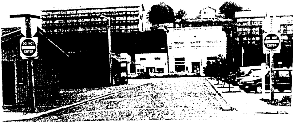
Figure 4: Alabama Street from the same vantage point as seen in Figure 3, in 1993. The fire was clearly a turning point for Bandon, and the town's building stock in the old commercial core has never returned to its pre-fire levels. Here we see clear evidence of Bandon's inability to recover its former commercial vitality from the 1940s to the present. The Masonic Temple in the background, which now houses art galleries, was one of the few structures to survive the fire. The motels on the bluff were built in the 1980s.
