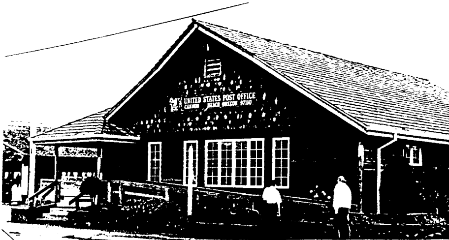
Figure 50: The Cannon Beach Post Office on Hemlock Street, the product of a remodel design in which Ray Watkins participated. The structure had been a plumbing and hardware shop with painted clapboard exterior façade prior through the 1960s. The structure was renovated in the late 1970s, with a combination of influences. The unpainted clapboard exterior suggests a local commercial influence, the accentuated front-gabled appearance, rough roof shingles, and hipped overhang suggest strong residential influences, while the unpainted decorative shingling and white-painted trim may be viewed as evidence of a New England influence. Fixed benches and flower boxes have been built into the native rockwork.
