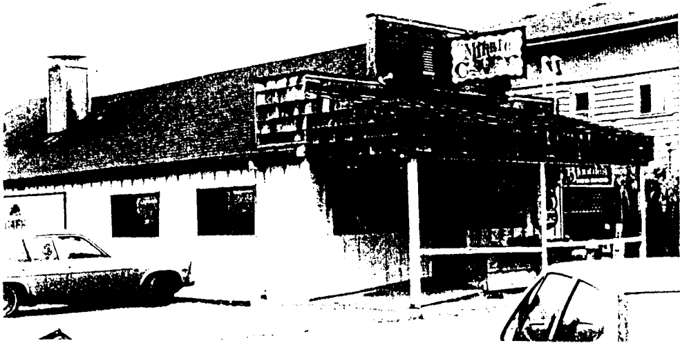
Figure 19: The Minute Cafe on Second Street. The façade is a 1980s addition, while the original building dates from the 1940s. Prior to the 1980s renovation, the building had a white painted rectangular façade with a suspended rectangular overhang. This façade features unpainted clapboard and rough shingles, while the overhang - though not an 'Oregon barn' style - is in a sloped style, with three-dimensional faces. This style lacks commercial precedents on the coast, but bears a remote resemblance to residential overhang styles. Note the flower box, and the use of an antiquated font on the sign text.
