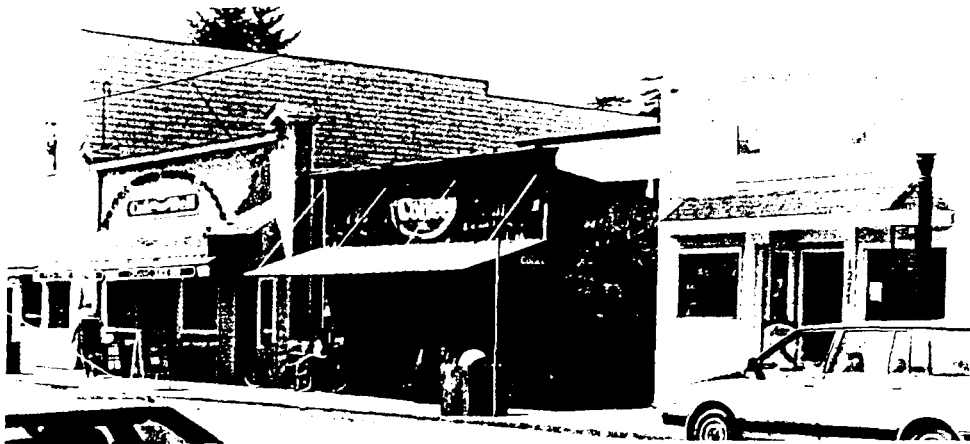
Figure 32: Three storefronts on the north side of Bay Street, in refurbished structures that house a cafe, coffee shop, and yogurt shop. The center structure, refurbished in the late 1970s, has been modified with a rough shingle exterior and a rectangular overhang. The other two shops, refurbished since the early 1980s, have been dressed up with freshly painted clapboard exteriors and somewhat non-traditional overhangs. The yogurt shop has gained a residential 'Oregon barn' overhang, which is scarcely broad enough to provide protection from the weather. Seating areas are placed at the exteriors of each of these businesses.
