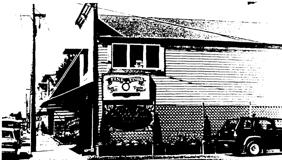
Figure 34: A Maple Street building dating from the 1890s, which was refurbished in the 1980s. This is the structure housing a bakery in Figure 26. The remodeling project involved the adding of fresh clapboard and overhangs, and the addition of lattice work and long flower boxes along the side of the building. The building housed a bakery for much of the first half of its history (Figure 26), and now houses a collectibles store, while flanked by a confectioner and an art gallery. The sign features the image of an antique pocket watch, and all text elements are in antiquated fonts.
