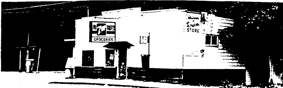
Figure 101: A small grocery store on Highway 4 on the outskirts of Port Alberni. (Map 19) This is a common look for rural Vancouver Island. Here we see that painted white horizontal clapboard still is used for commercial applications in less tourist-oriented settings. The diagnostic mnemonic cues are absent, while textual and logo signs are present, being more common on such thoroughfares.
