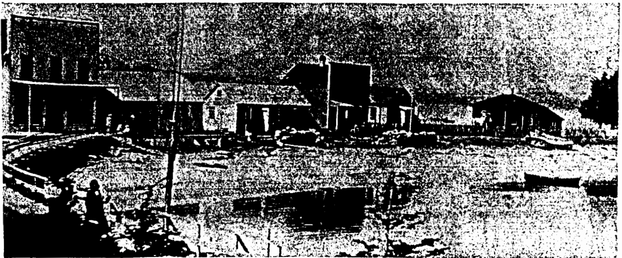
Figure 80: The village of Clayoquot, predecessor to contemporary Tofino, on the opposite shore, ca.1911. (Map 20) Commercial buildings are clearly suggested by rectangular façades with clapboard siding. Houses are side-gabled, or front-gabled with hipped roof Photo courtesy British Columbia Archives and Records Service. (Negative #F-495)
