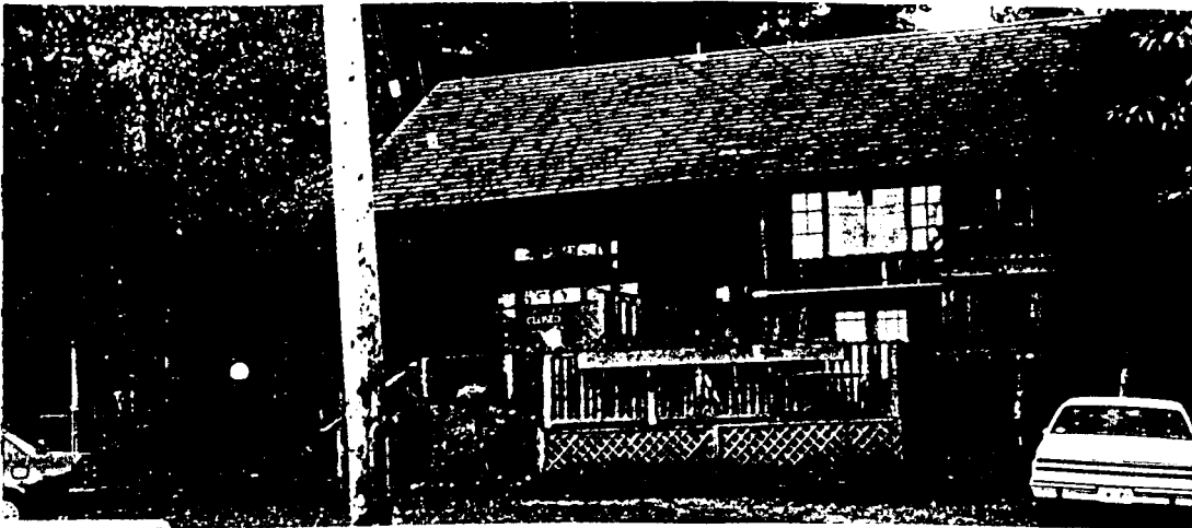
Figure 99: A restaurant on Campbell Street at the east end of Tofino, of 1980s construction. The structure is side-gabled, with a hipped roof extension, and an unfinished batten-and-board exterior. The door and small-paned windows are also natural wood, with a transparent finish. The appearance of this structure hints at both side-gabled residential buildings as well as industrial buildings. (Figure 84) The round windows may be considered suggestive of port hole windows. Though scarcely visible in this photo, flower boxes are placed around the front of the building.
