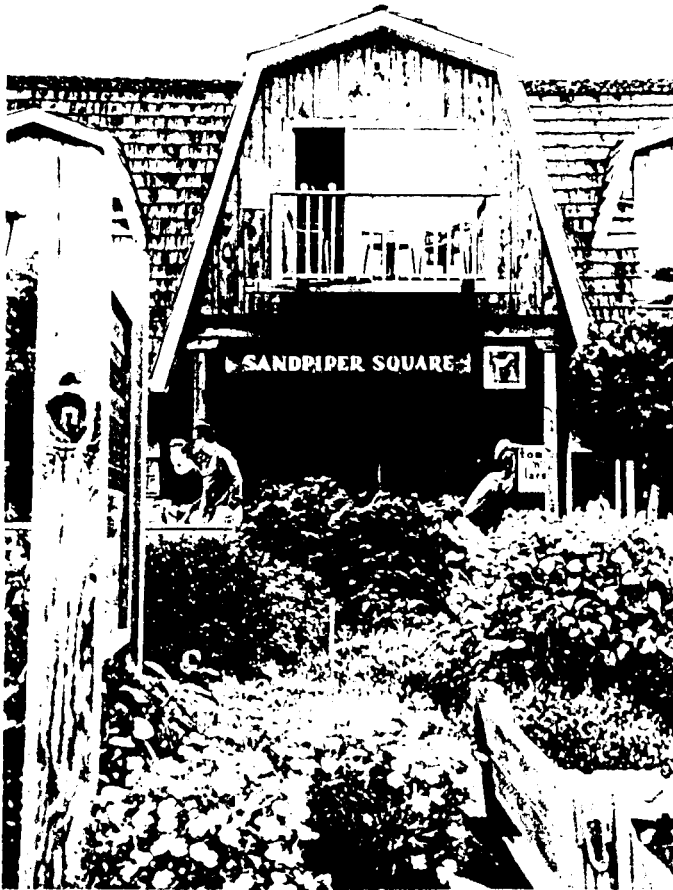
Figure 51: The central portion of Sandpiper Square, a collection of shops on Hemlock Street, in a building based on a Ray Watkins design. This structure, built in segments between 1968 and 1973, is based upon the look of New England coastal buildings, with gambrel roof and dormers; this design has no clear precedents on this coast. Still, the rough board-and-batten exterior and the rough shingled roof echo Northwest coast industrial and residential buildings. The foreground landscaping was built over a parking area in the 1980s; this area, designed by the son of artist Bill Steidel, features statues of herons, fixed flower boxes, and an assortment of benches. Note also the image of a sandpiper on the archway sign.
