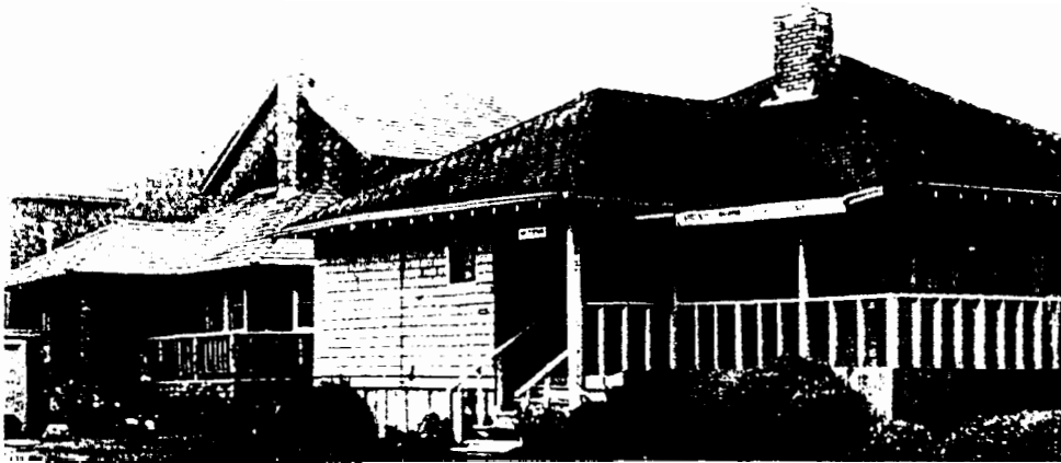
Figure 57: A residential example of the infusion of the New England look into Cannon Beach. These two ocean-front structures, on Pacific Street in the Tolovana Park district of Cannon Beach (Map 12), were almost identical prior to the renovation of the structure on the left. Immediately prior to the sale of this house, owners added a second story, replaced exterior painted shingles with unpainted shingles, shingled the deck skirt and support posts, replaced tar paper roof shingles with unpainted wooden shingles, and painted the trim white, among other things.
