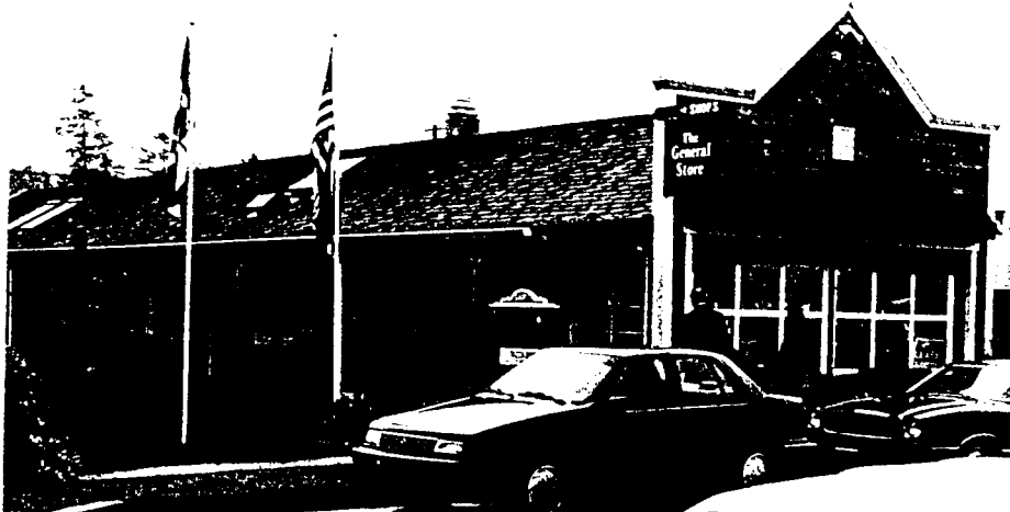
Figure 56: The General Store, a collection of shops on Hemlock Street. remodeled in 1992. This structure - of 1940s construction - housed simple apartments, clad in white painted clapboard. In the renovation project, investors added the unpainted clapboard façade, the overhang over shop entrances, large windows with implied small panes, benches, flower boxes, signs, and landscaping with U.S. and Canadian flags. On the street face, we see a shallow overhang with no protective value, under which has been placed a stylized harpoon.
