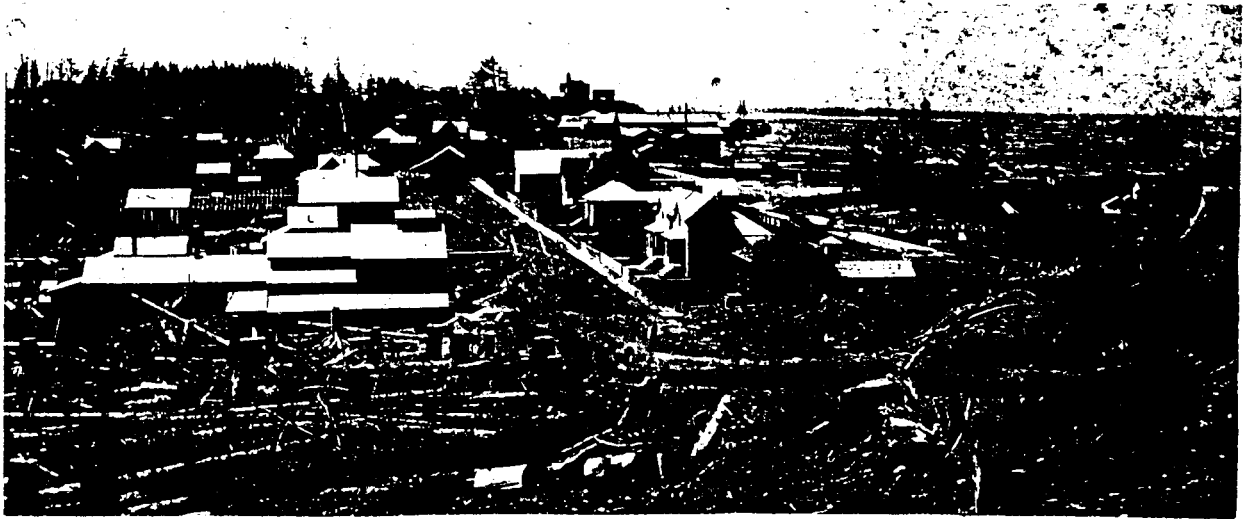
Figure 1: Bandon in the late 1890s, looking west down Third Street, then the main street of the town. 36 Most one-story houses have hipped roofs, while the two-story houses have gabled roofs. The two gothic style homes on the right side of the street have enclosed 'Oregon barn' type entryways, though complete 'Oregon barn' style homes - one-story and front gabled - are absent. All visible houses are clad in painted clapboard. Only storage sheds - such as the shed behind the house in the foreground right, and the mill outbuildings on the left - are clad in rough shingles. Only industrial structures, such as the main buildings of the sawmill and foundry, left foreground, have vertical, unpainted board-and-batten exteriors. Commercial functions, not seen here, are clustered near the industrial waterfront, with rectangular, painted white clapboard façades. Photo (Negative #63) courtesy Coquille River Pioneer Museum.
