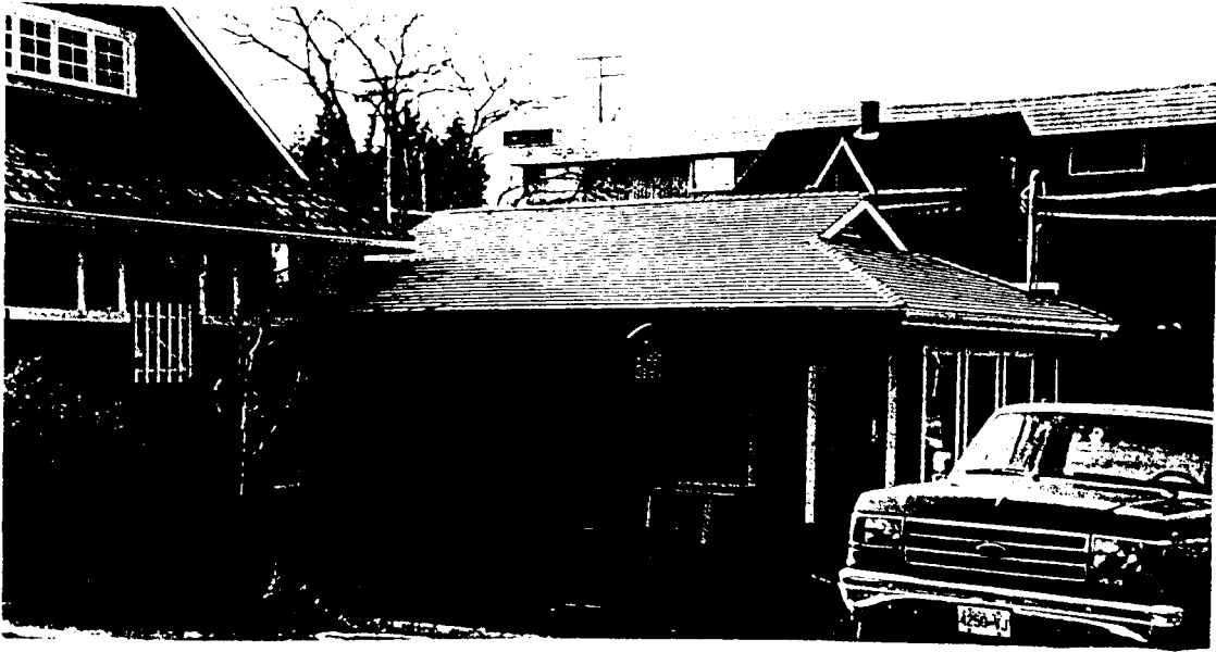
Figure 93: The Village Gallery, a Main Street art shop, shortly after its construction in 1993. The low-pitched gable-on-hip residential style construction provides an 'Oregon barn' echo to the residential building onto which the Gallery was built. The residence is from the period when Tofino was primarily a Norwegian resource settlement. (cf. Figure 83) The Gallery has an unpainted shingle exterior, as of yet unplanted flower boxes, and a sign which features a windsock kite, all features reminiscent of the American towns in this study.
