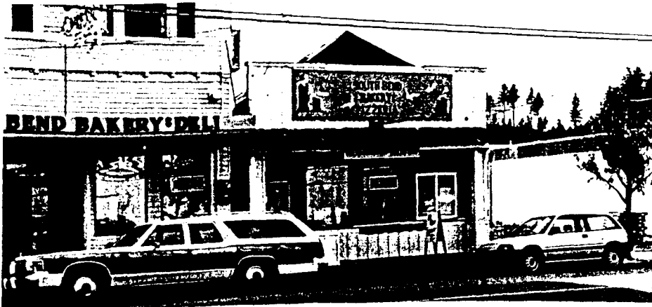
Figure 76: A site on Highway 101 with a telling history, this commercial structure is a remodelled residential building which had replaced a pre-existing commercial structure. The value of the space for commercial uses declined after the 1920s, but has gradually increased following the 1950s. The building now consists of a hipped-roof residential building, with attached painted white façade, a shallow shingled overhang with no protective value, and horizontal unpainted boards around the entry. Note the gull and pier motif on the sign.
