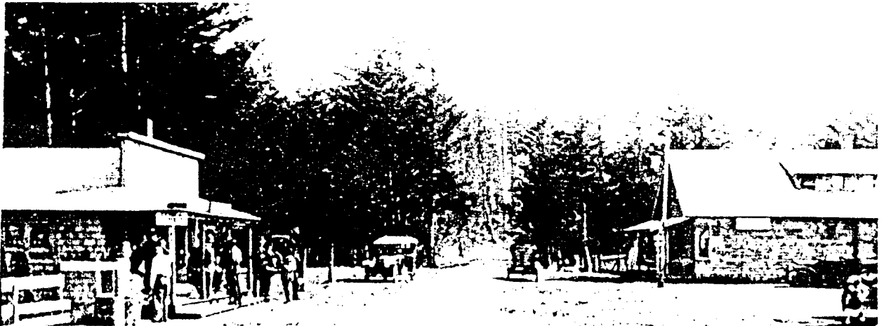
Figure 42: Downtown Cannon Beach, looking south on Hemlock Street, in the late teens or early 1920s. The buildings date from the World War I-era, and were likely built to service Spruce camp labor. One - a newspaper shop and post office - features a rectangular façade, while the other, a combined residence, storage area, and general store, is front-gabled without façade. Both structures feature overhangs and unpainted shingles. Immediately after this time, in the photographic record we find both structures painted. Only small, textual signs are present.
