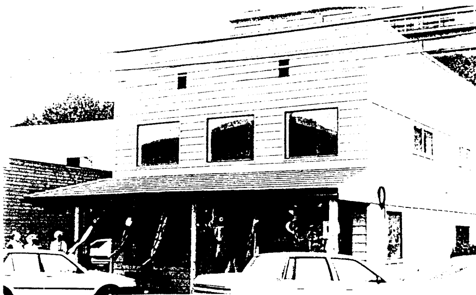
Figure 16: Grotto Gifts on Bandon's Second Street. The building is of early 1980s construction, and shows the influence of other historical commercial structures of the area, with painted vertical clapboard on its rectangular face. The overhang is something of a hybrid, wrapped around two sides of the building; the hipped construction may possibly be viewed as an 'Oregon barn' derivative. Note the windsocks hanging in a row on the eave, and the flower box. The gift shop's sign, around the corner from this photo angle, features an ocean scene with sea gulls.
