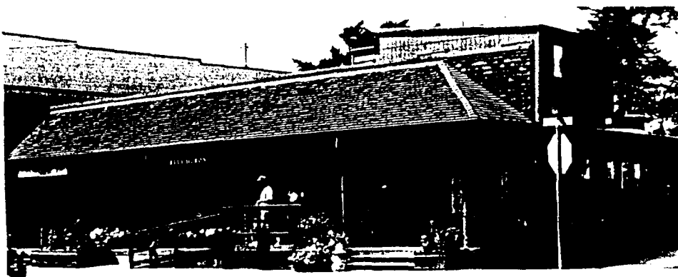
Figure 38: A building on Bay Street, of late 1980s or early 1990s construction, housing galleries and gift shops. This building's design is an interesting adaptation, structurally no different from other boxy commercial mini-malls of the North American commercial urban vernacular. Yet the façade shows a clear influence of a hipped 'Oregon barn' overhang and a rectangular façade with shingles. The overhang, usually only covering one entrance, has been expanded to enclose all store entries in this complex. The 'Oregon barn' overhang has little protective value, as it has been attached as an expressive feature onto an unrelated structural overhang. The combination of façade, shingles, and hipped overhang, of course, was not seen until the 1970s. It is now a common tourist-oriented hybrid. Note also flower boxes, and - in the shadows - benches on the porch, and windsocks in a row, hanging from the side eave on the right hand side of the building.
