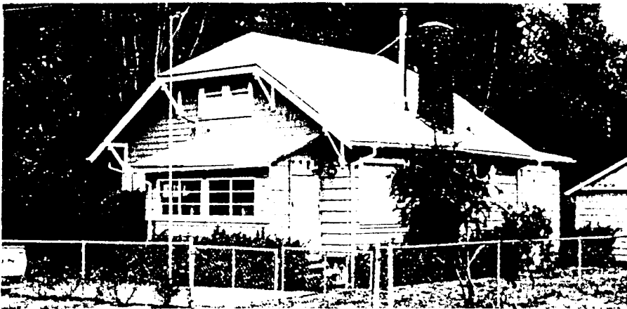
Figure 41: A house on Larch Street north of Ecola Creek, dating from roughly 1910. (Map 12) 45 This structure was a farmhouse during the brief agricultural phase in Cannon Beach. The hip-on gable, front-gabled roofline was common in the area at the time of construction, as was the use of local beach rocks and sand for chimney construction. Painted shingle exteriors, as seen here, were also common on houses of this era. Though not clear in this photo, this house was built on pilings in a filled corner of a large marsh.
