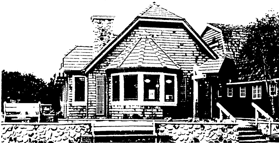
Figure 48: A Hemlock Street ice cream shop of 1993 construction, showing the clear impress of vernacular house styles of the area. This Ray Watkins design utilizes the front-gabled hip-on-gable style of pre-1930s structures with shingled exterior, and native rockwork. Unlike the residential examples of this style, the shingles are not painted. (cf. Figure 41) This structure, like many other recent commercial buildings, includes benches, and flower pots - both free-standing and fixed - in its initial construction.
