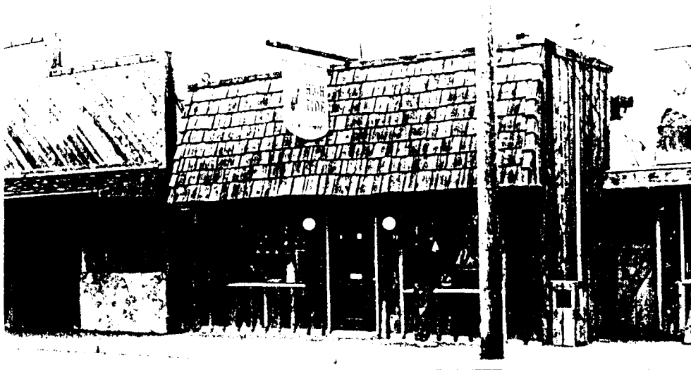
Figure 14: The High Tide Gift Shop on Second Street. This façade replaced a white painted clapboard façade during the 1970s, when this building housed a tavern. The rough shingles and board-and-batten exterior were not found in commercial applications prior to this time. Note the blue heron image on the Shop's sign.
