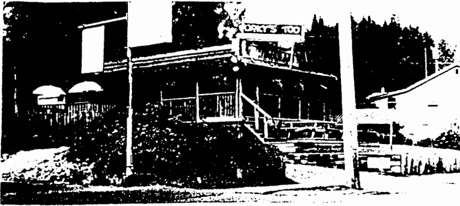
Figure 110: Porkey's Too Restaurant, in a Peninsula Road building of 1980s construction. The structure clearly shows influences of historical commercial structures with rectangular façades, though the unfinished wood siding and porch supports, as well as the low-pitched hipped overhang are from industrial and residential precedents. Note the hanging flower pots placed around the porch.
