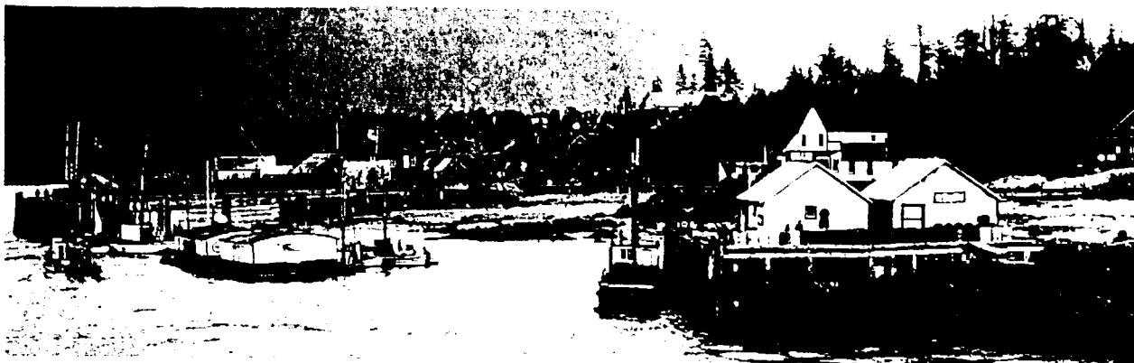
Figure 84: The Tofino waterfront of the 1930s. By this time, Tofino had surpassed Clayoquot as the area's commercial core. White painted clapboard is still used for most commercial buildings, though by this time, the western rectangular façade is not being reproduced. Only storage sheds, as seen center photo, and other industrial facilities are constructed with unpainted board exteriors. Note the 'Oregon barn' style overhang on the house in the right foreground. Photo courtesy British Columbia Archives and Records Service. (Negative #D-1341)
