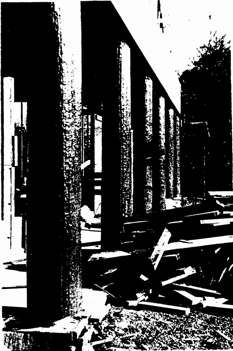
Figure 95: The front of the Himwitsa Center, on the corner of Main and First Streets, under construction during 1993. These posts have been specially hand-adzed, and coated with a transparent finish, to provide the appearance of tribal building styles on an otherwise ambiguous Canadian urban vernacular form.
