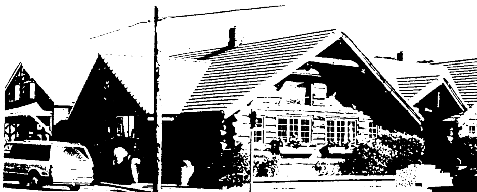
Figure 52: Morris' Fireside Restaurant, on the corner of Hemlock and Second Streets. This structure was built in the early 1980s, on the site of the structure shown in Figure 43. While still maintaining the log construction, this structure suggests a more complex lodge design. This structure features windows with inserts which create the effect of small panes, native rockwork, and built-in flower boxes and benches. Note the 'Oregon barn' design of the gift shop in the left background.
