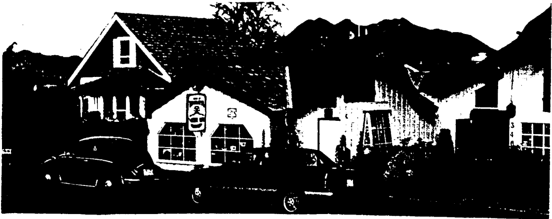
Figure 91: The House of Himwitsa, a Northwest coast native art and trinket shop on Campbell Street, dating from the 1980s. The building style appears to be a whimsical fusion of residential and barn elements. The sign features a stylized tribal image of a human and a seal. Three vertical logs - suggesting piers - have been placed in front of the entryway.
