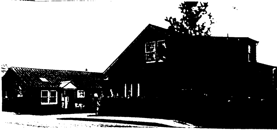
Figure 59: The Blue Gull Motel on Hemlock Street in mid town Cannon Beach. (Map 12) This older motel building, dating from the 1950s(?), was refurbished in the late 1980s. After this time, the side-gabled motel structure has had a distinctly residential face on its street side, with adapted window placement and added overhang. The overhang provides no protective value for pedestrians, as all entrances are still on the building's sides. The Motel's sign, scarcely visible on the right edge of the photo, features the image of a sea gull.
