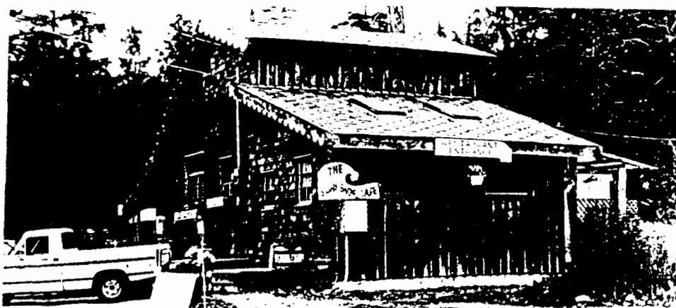
Figure 103: The Surf Side Cafe and Surf Shop, along the roadside on Highway 4, south of Tofino. (Map 20) This salt box and shed style of building is an anomaly on the west coast of Vancouver Island. The whimsical irregular shingling - on the street-side face only - reflects local residential styles, while an industrially-influenced board-and-batten exterior has been built on the other faces. Flower pots are plentiful, primarily placed on the street face. The signs are in the images of waves, while bamboo torches frame a large flower pot, adorned here with a temporary sign.
