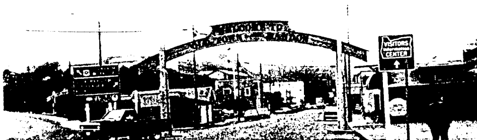
Figure 12: One of Bandon's arches in 1993, built in the 1980s at the Highway entrance to Second Street, one block east of the location of the historical arch. This arch resembles the historic arch, but, like the rest of the town, now has a more rustic, wooden appearance. The arch is supported by vertical poles of different heights, which are lashed together with heavy rope, suggesting piers.
