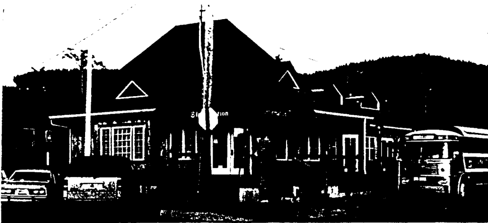
Figure 65: The Cannon Beach Chamber of Commerce building on the corner of Second and Spruce Streets. This building, of late 1980s construction, suggests a strong residential influence. The board-and-batten exterior reflects the town's historical industrial building, while the white painted trim and implied small-pane windows reflect the town's neo-New England look. The exterior of the building is adorned by sculptures by local artists of wildlife and tribal images. Flower boxes and benches are built in to the exterior of the building.
