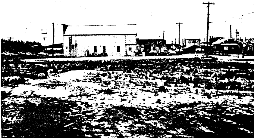
No. 12, Fig. (vi) Vacant lot Eliot St.
