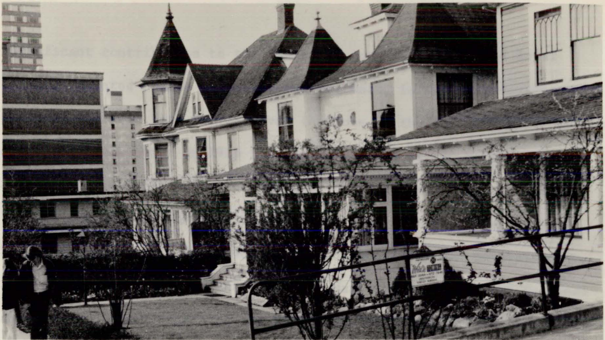
Plate 14: Old Houses in Vancouver's West End. - The West End still contains some fine old houses such as these on Robson Street which have been privately restored in recent years.
