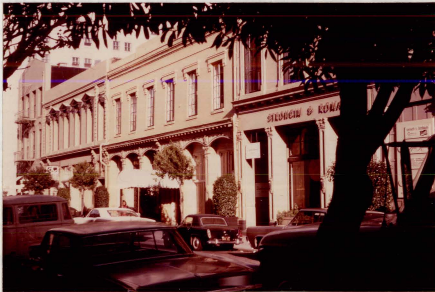
Plate 5: The Jackson Square district of San Francisco.- This was one of the few areas of San Francisco to survive the 1906 earthquake and fire, and hence it comprises one of the greatest concentrations of early San Francisco architecture. The area went through a long decline, but was rediscovered and restored in the 1950's, providing one of the first instances of historic district preservation activity in a young North American city.
