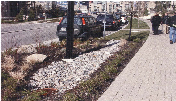
Figure 8.1: Design Boulevards to Improve Storm Water Management
