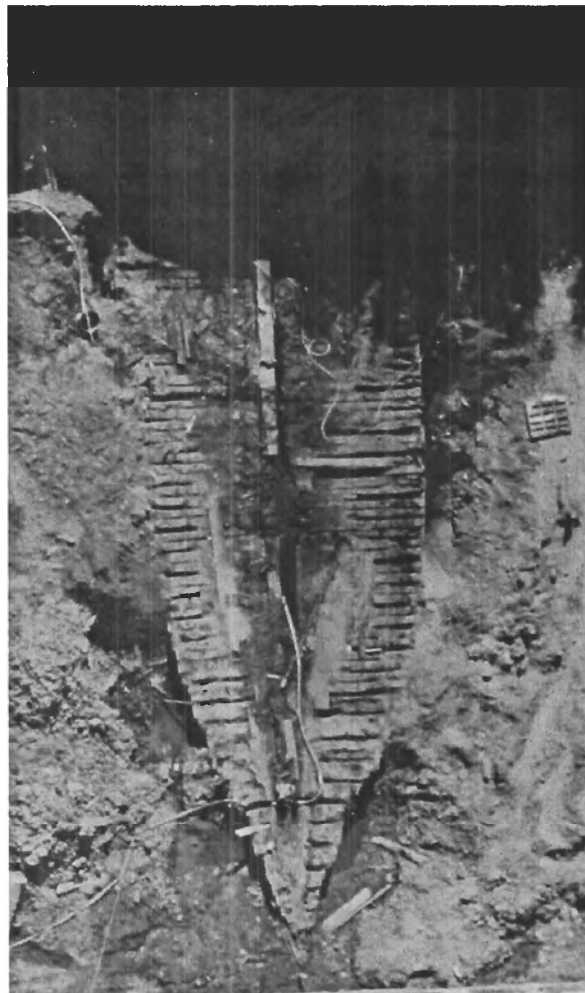
Figure 7: Elevated view of Niantic as exposed in May 1978. The pointed end of the hull is the stern; the bow is buried beneath the adjacent Redwood Park. San Francisco Maritime National Historical Park, National Park Service Niantic Excavation photographs, P88-032 and P84-008.
