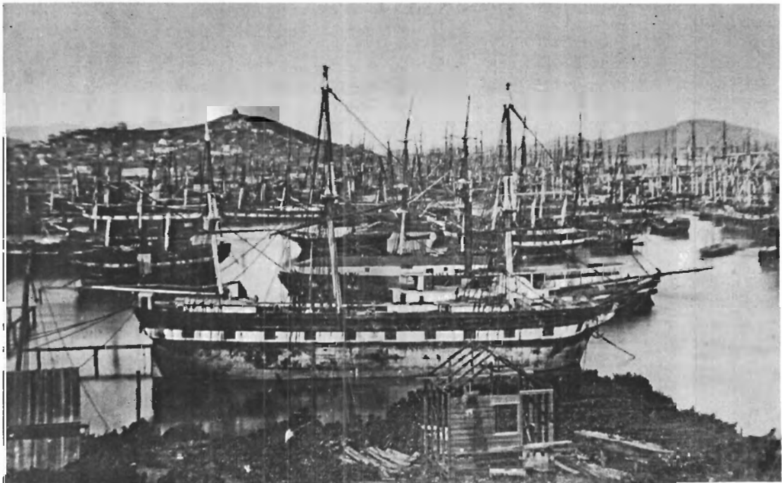
Figure 5: This view of Gold Rush ships about to be scrapped at Rincon Point dates to 1853 and is part of a larger panorama by William Shew. Of particular interest is the storeship behind the hulk in the foreground. The weather deck supports a single story barn much like General Harrison's . San Francisco Maritime National Historic Park, J. Porter Shaw Library A11.4, 528-c n.
