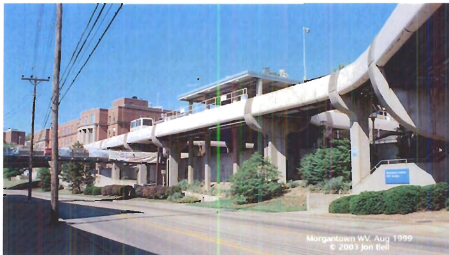
Figure 2.1 Photos of Morgantown PRT System
