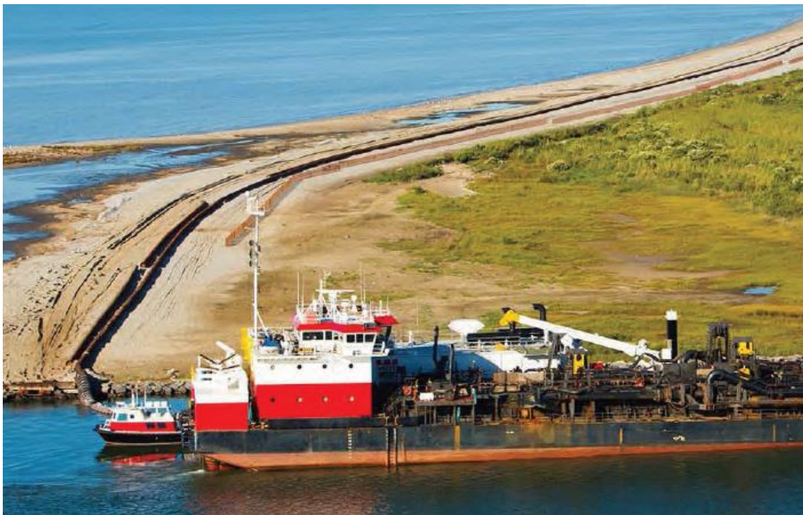
Figure 15: Dredge boat and sediment pipeline; Louisiana CPRA, 2017.
