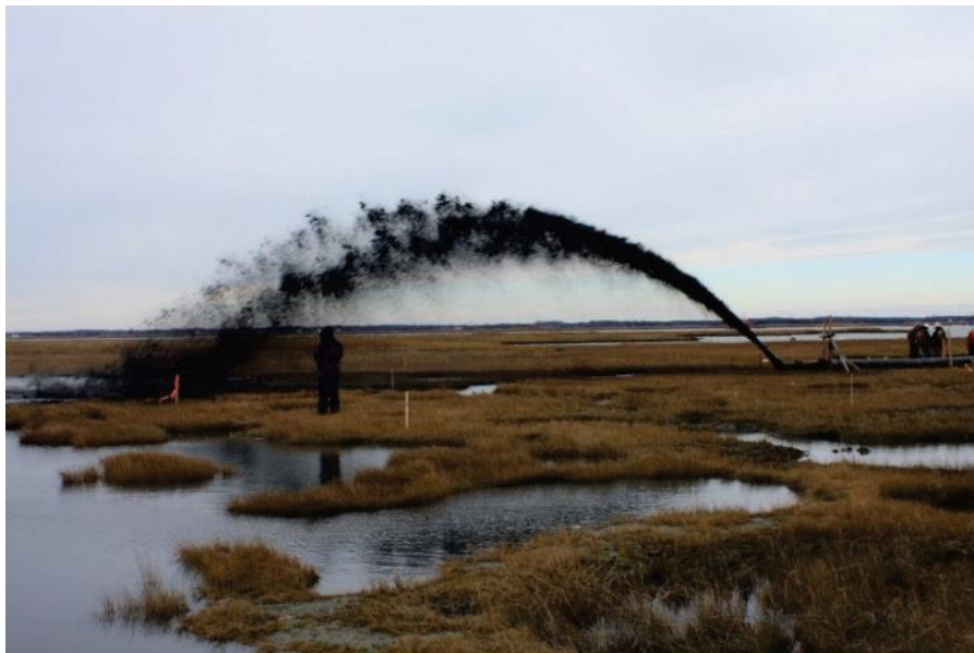
Figure 13: Thin layer placement of sediment. Photo credit: Tim Welp; USACE, 2019.
