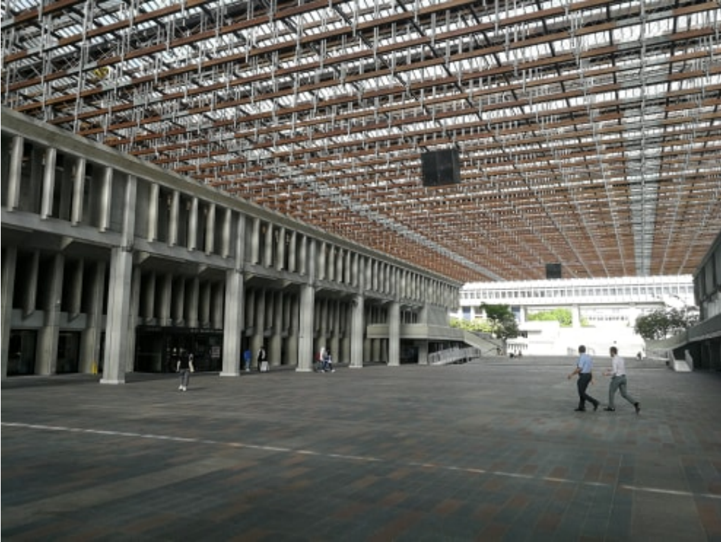
Figure 24) Newly paved Convocation Mall after renewal project (Author)
