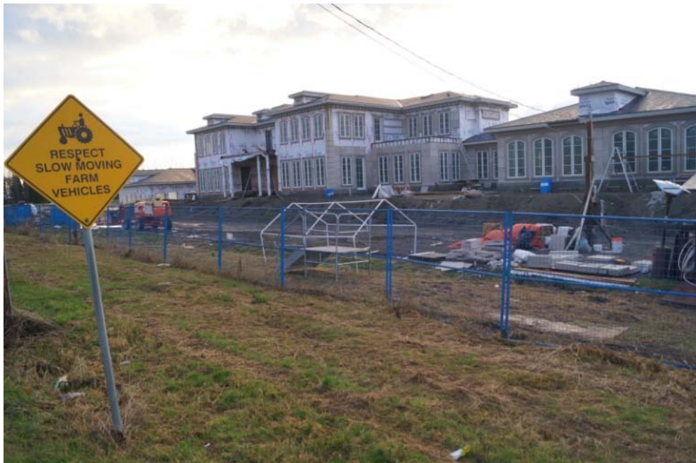
Figure 1.5 A 2,050 m 2 ALR Dwelling Under Construction in 2017, South of Steveston Highway
