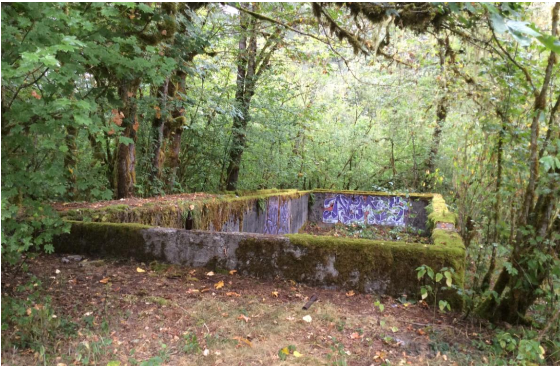
Figure 42. Overview of concrete pool remains. Photo facing northwest.
