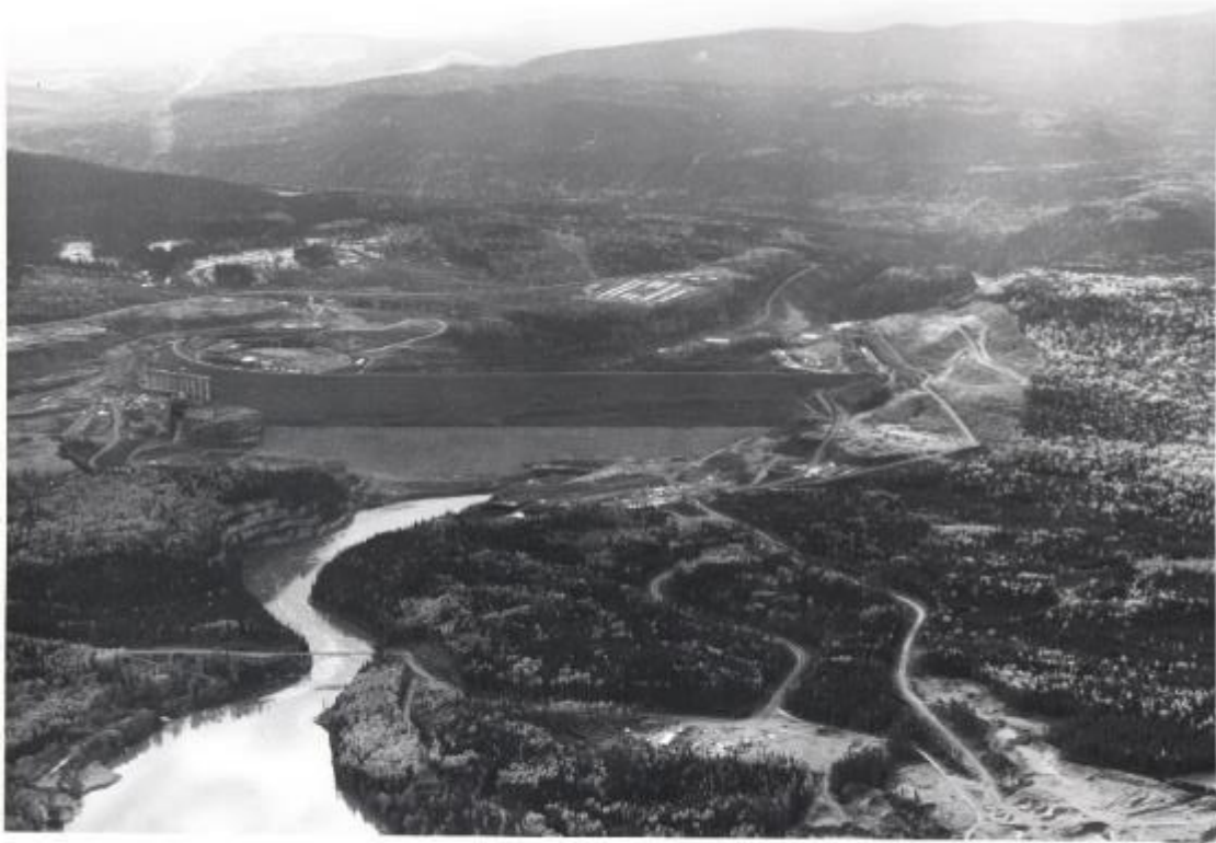
Aerial view of W.A.C. Bennett Dam from upstream, Spillway Complex on the right, - Penstock Intake Structures on the left, #046670
