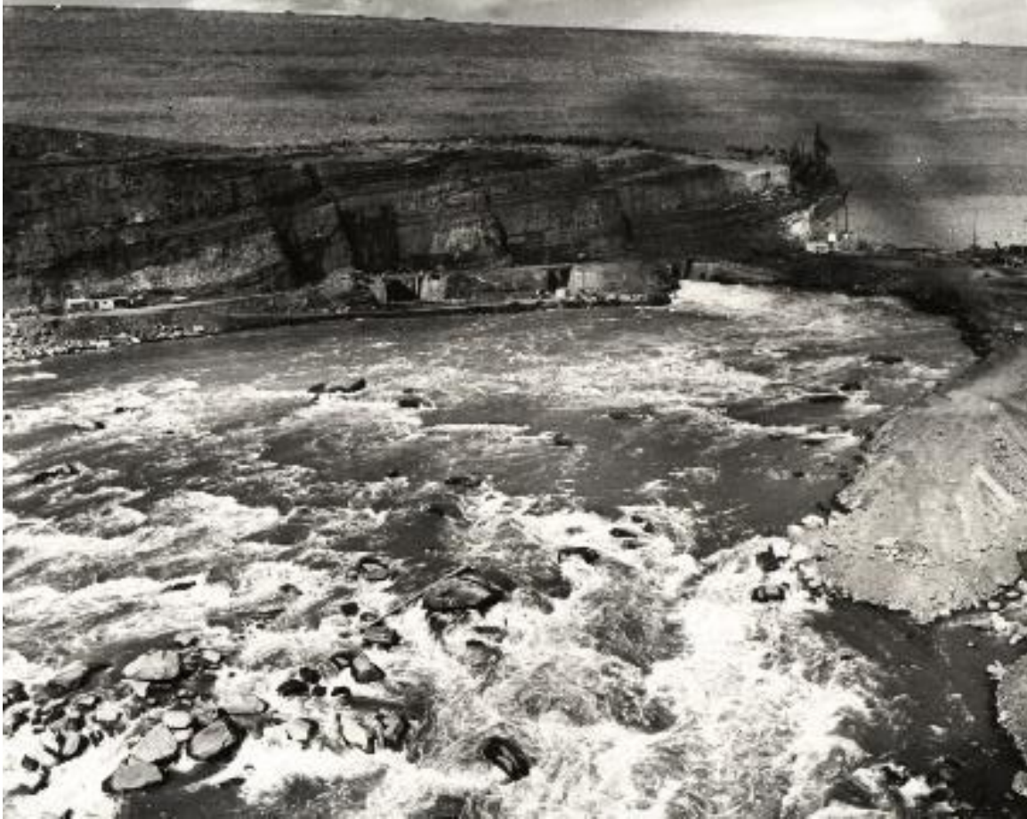
Figure 22. Bennett Dam during construction. Archival Image 1981.BEN.015 Hudson's Hope Museum and Archives
