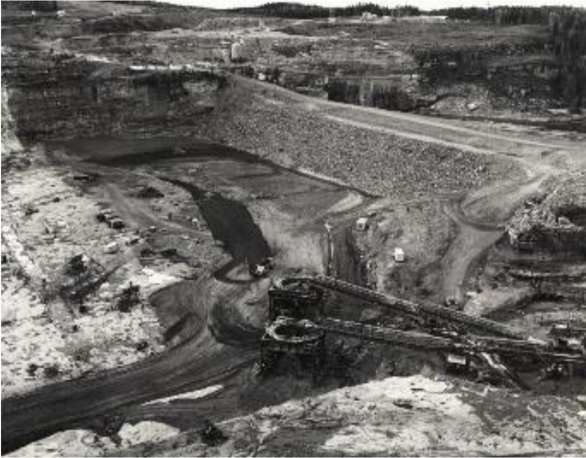
Figure 23. W.A.C. Bennett Dam During Construction. Archival Image 1981.BEN.004. Hudson's Hope Museum and Archives
