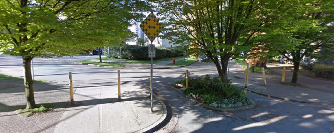
Pendrell and Bidwell traffic diversion intersection: Lack of marked pedestrian crossing
