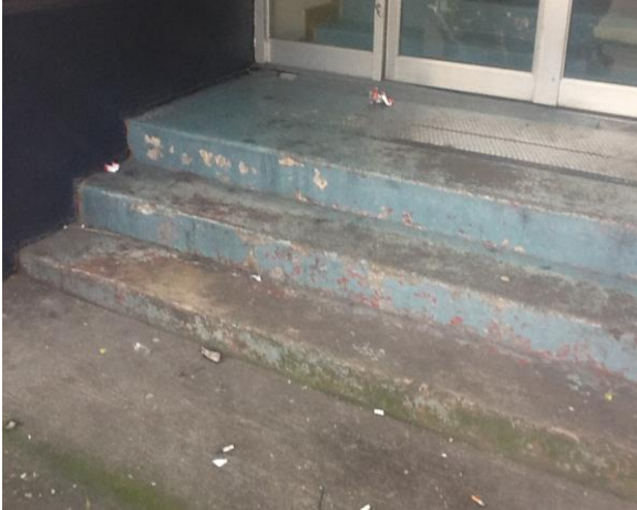
Inaccessible shop, Denman and Robson
