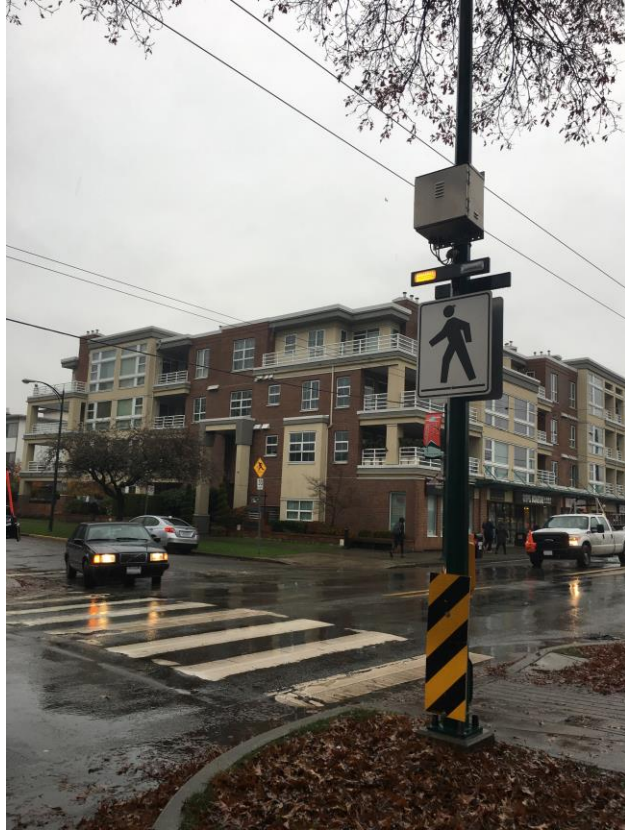
Figure 5.16. Crosswalk Design. This crosswalk consisted of several design features that participants said made them feel safe when crossing the road, namely: flashing lights, audible beeping, a zebra design, and adequate signage.
