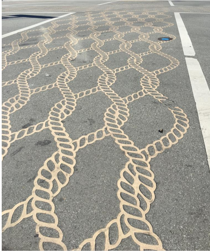
Figure 5.19. Rope Design. The rope design in this scramble crossing was identified as overwhelming for the participant, making it challenging for them to navigate this crosswalk independently.
