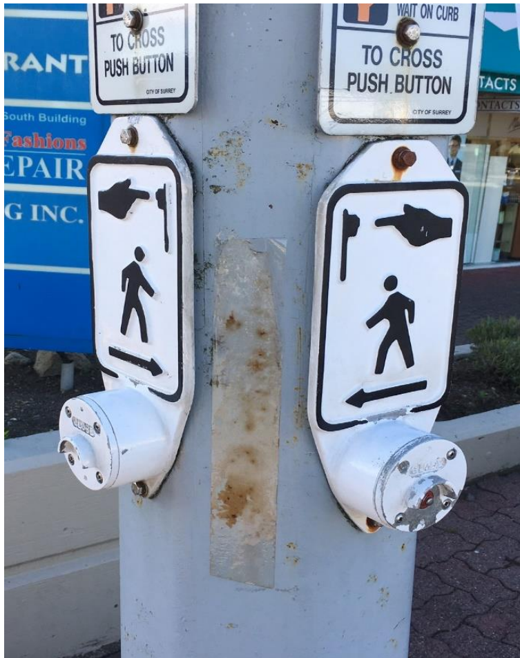
Figure 5.17. Crosswalk Buttons. These buttons appeared on the same pole. The data reveals that this can be confusing for some people with dementia.
