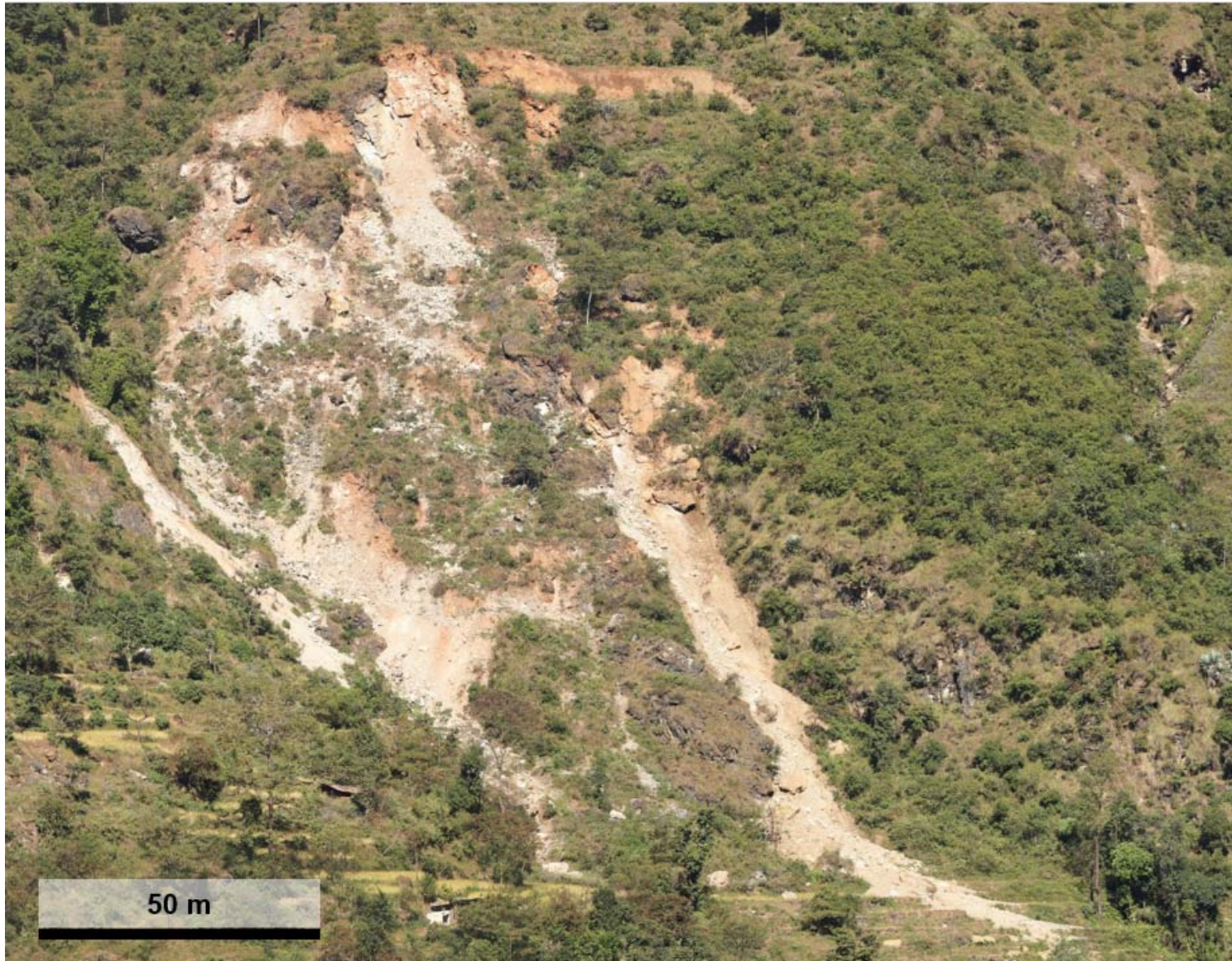
Figure H 4. Composite image of failure west of TLR as shown in Figure 5-2(a) in main body of thesis. Created from photographs collected November 6, 2016 looking north-west.
