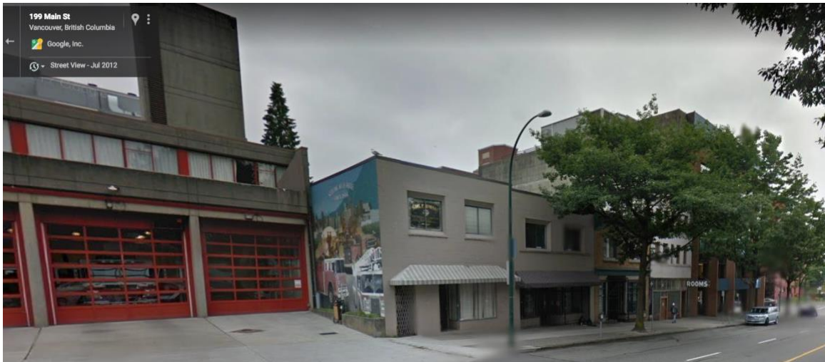
Figure 3 Fire Hall No.2 in the Downtown Eastside sits next to vacant retail storefronts and Single Room Occupancy Hotel (SRO) and mixed-use office with ground floor retail. At the end of the block is a rail overpass to the waterfront and Port of Vancouver
