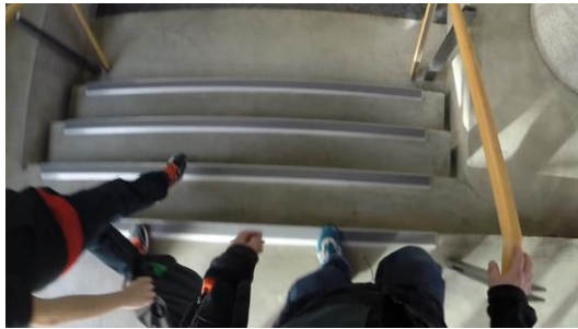
Figure 2.2. A short flight of stairs between floor and stair landing
