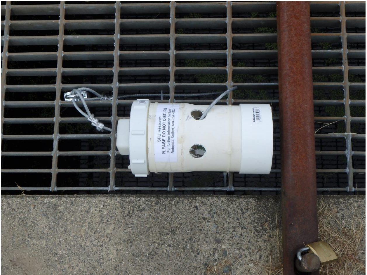
Figure A2. Cameras were placed inside a protective housing like the one pictured here and locked to flood box accessory structures (e.g. grates and railings). At this site and several others, floodgates are located beneath a grate. The camera lens was positioned to focus on the gate(s) through holes in the grate.
