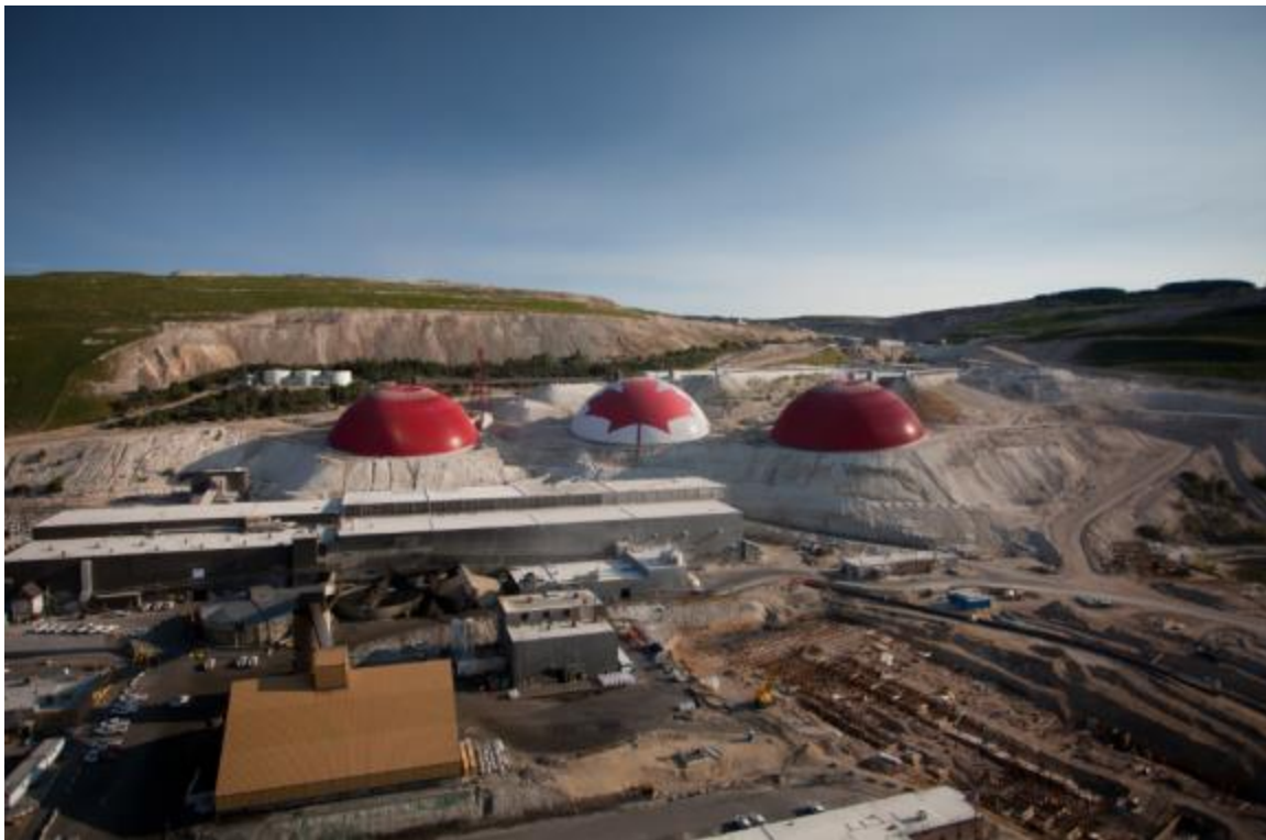
Figure 1 - View of Teck Highland Valley Concentrator Complex and Ore Storage Covers
