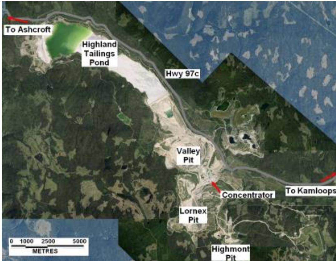
Figure 3 - Highland Tailings Pond
