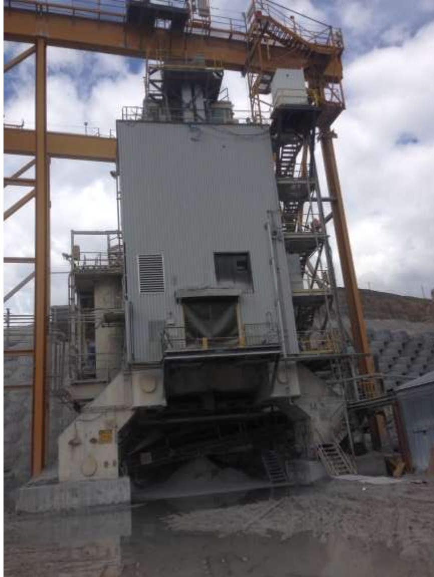
Figure 2 Crusher #5 Superstructure and Gantry Crane (by Author)
