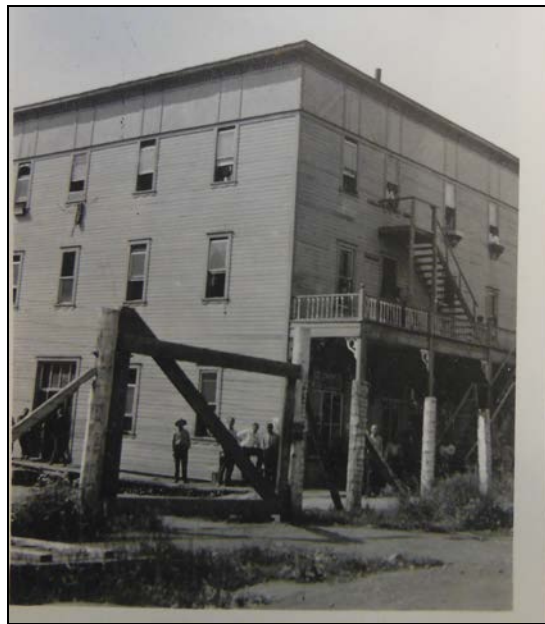
Figure 6.5. Morrissey Hotel, also known as the “Big Building” and later the “Slav Compound”
