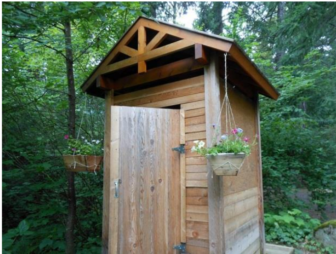
Figure 13: Campground Outhouse (Photo: Robin Trethewey, 2013 with permission)
