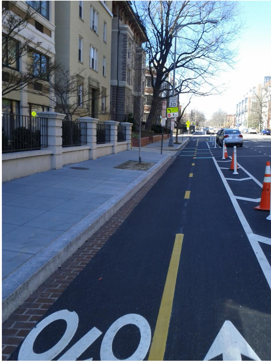
Figure C.1. 15 th St. Bike Lane
