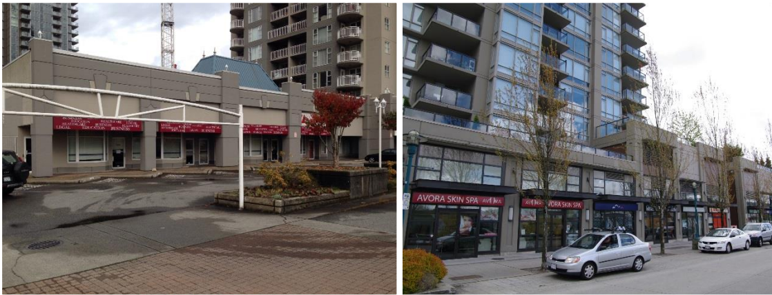
Figure 13 Pre-2004 podium with angel parking (left); post-2004 retail podium with residential above (right)
