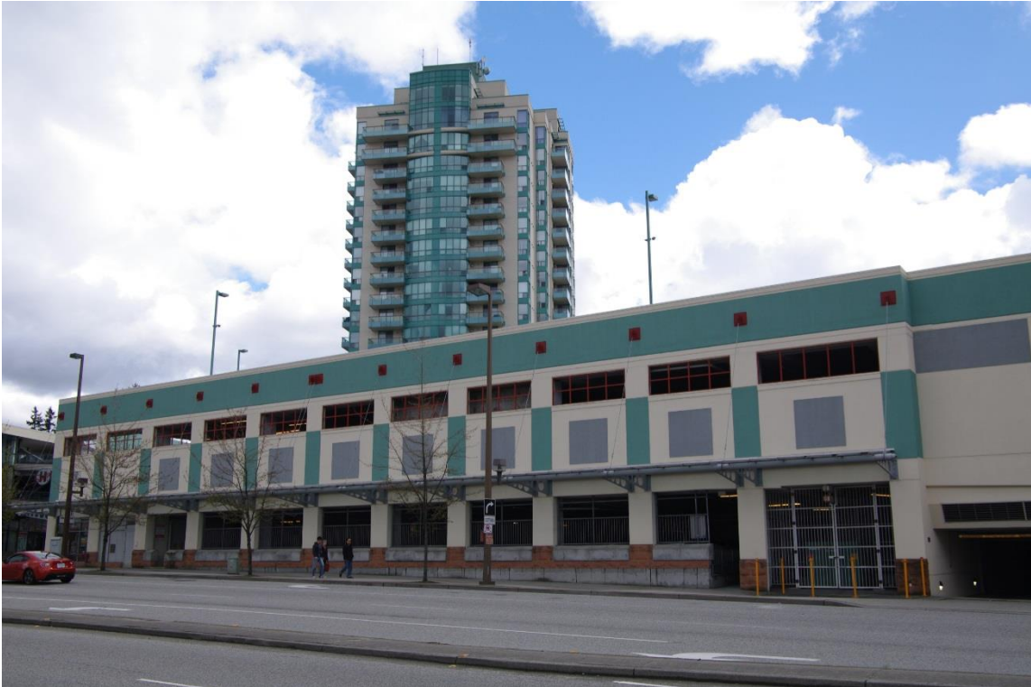
Figure 4 Henderson Centre: 1990 to 2004 Era – 1163 Pinetree Way, Coquitlam
