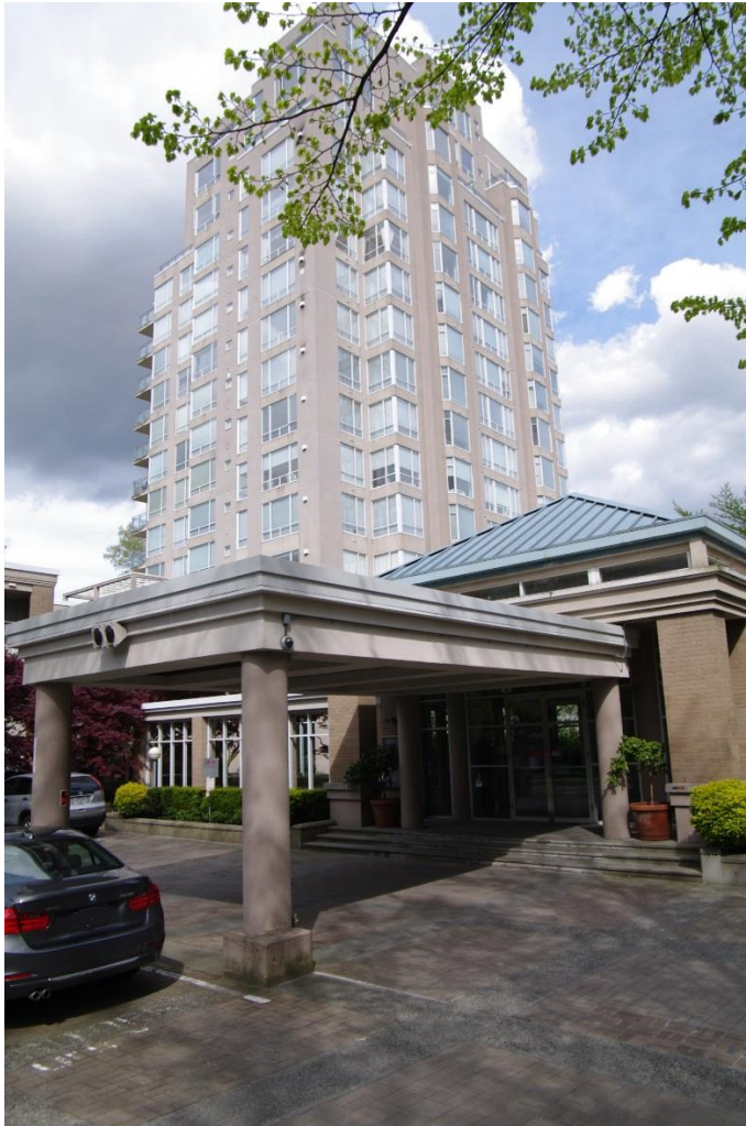
Figure 6 The Cambridge Gardens: 2668 Ash Street, Vancouver - Built 1990
