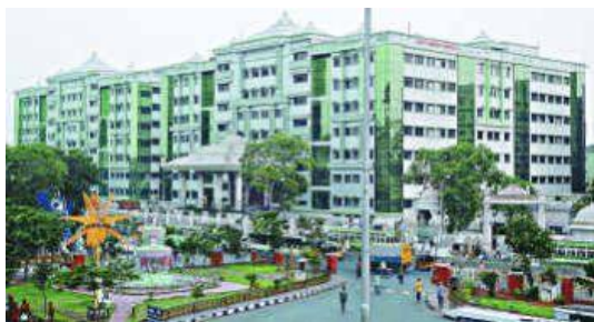
FIGURE 1 – GOVERNMENT GENERAL HOSPITAL EXTERIOR (CRED. GANESAN, 2005)
