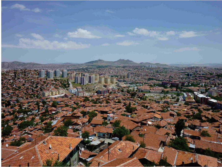
Figure 1. Towers in the distance foreshadowing the future for many of the remaining gecekondus
