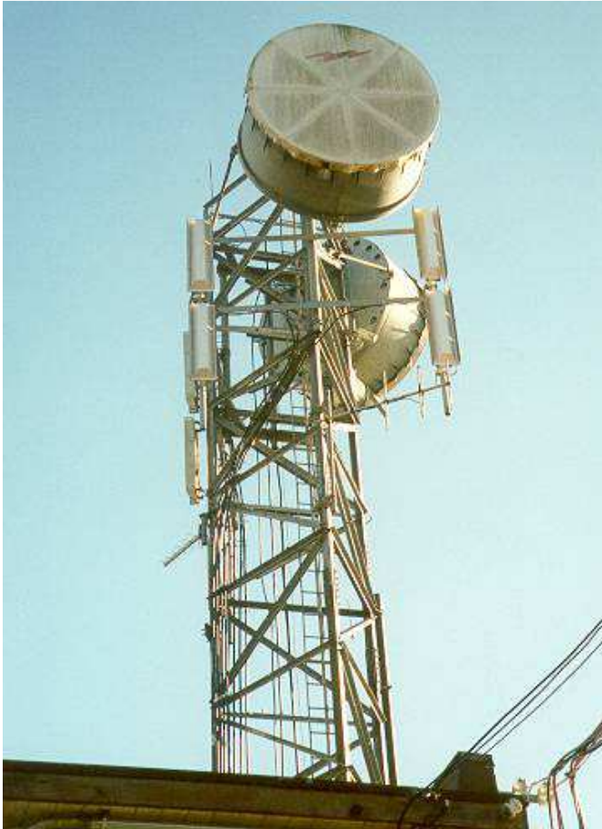
Figure 3: A Lattice Tower in North Vancouver, BC
