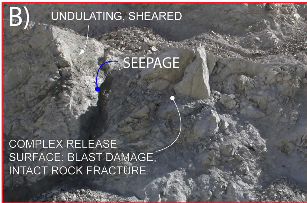
Figure 6 - 4: Bench-scale wedge failure in Design Sector 2, with an undulating J5 sliding surface with groundwater seepage; release occurs on complex blast-damaged and weathered surface with evidence of intact rock fracture.
