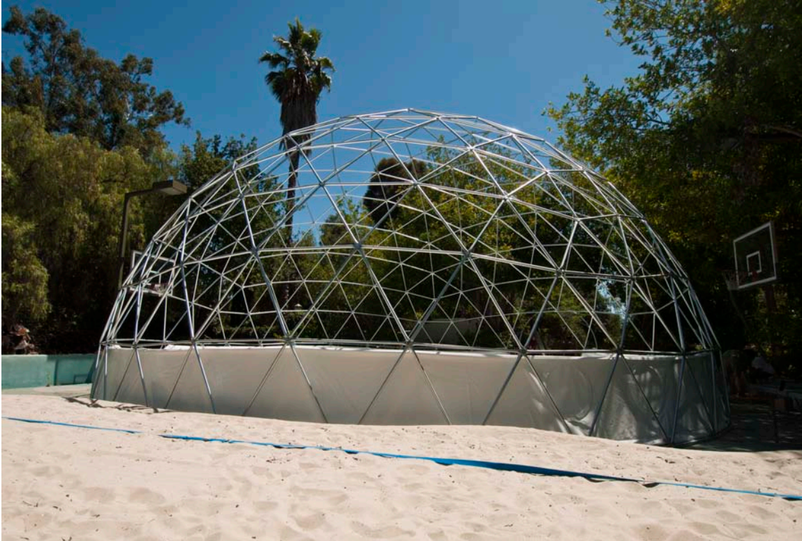
Figure 12. Geodesic Dome Lattice (pre-build)
