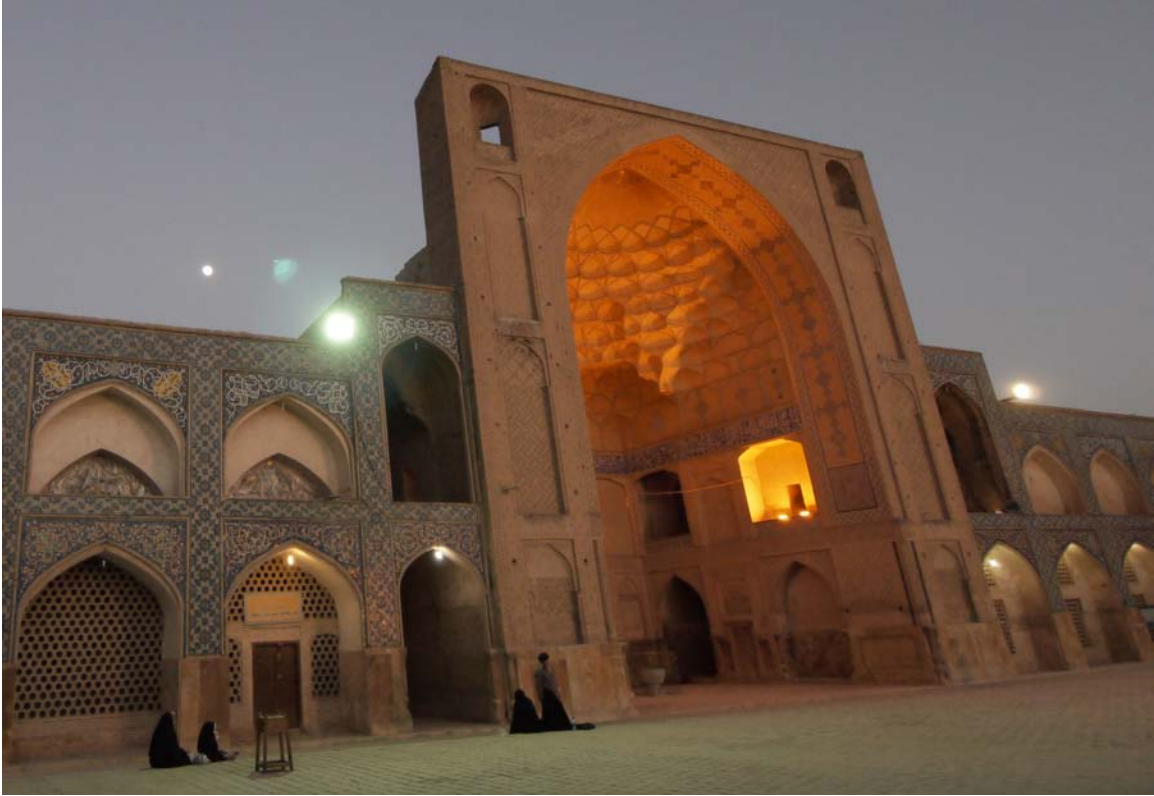
Figure 4. Partial Exterior of Jami Mosque (Isfahan, Iran)
