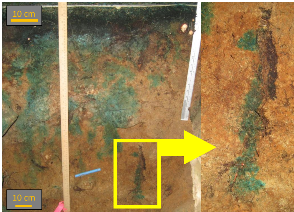
Figure 3.14: a) Flow along a decayed root in profile 5 of the TIE, where the maximum infiltration occurred at 85 cm (outlined in orange). Scale distorted vertically. b) Close up of infiltration through decayed root and fine roots, into matrix below.
