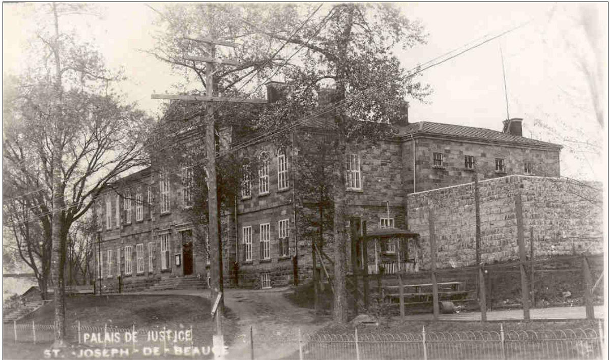
Illustration 2. The Palais de Justice in St-Joseph, undated picture. The high wall on the right surrounded the prisoners' exercise area. ASPB: PR129-1-3-12-STJO-84
