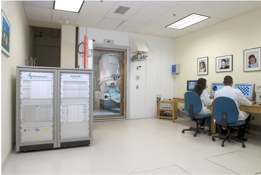
Figure 3.1: CTF Installation at Down Syndrome Research Foundation, Burnaby, BC, Canada
