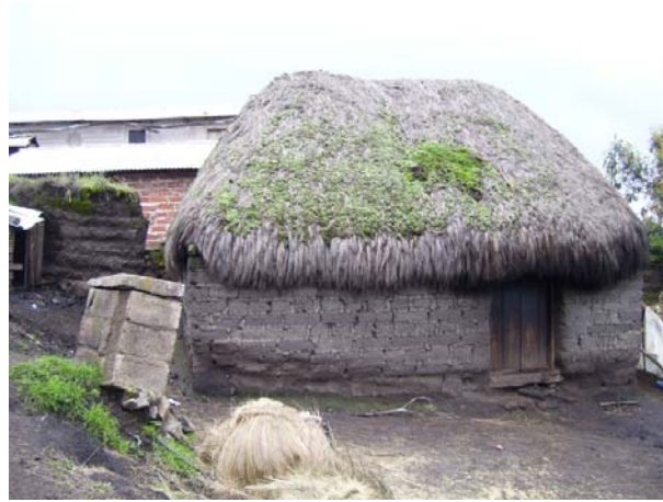
Figure 33. House with mix of adobe walls and thatched roofs construction, Cruz Loma, Sicalpa
