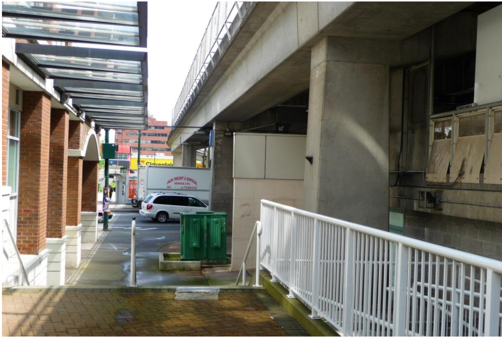
Figure 14 – Impermeable station structure and newer buildings along Main Street, west side, May 31 2011 (Source: © A. Jones)
