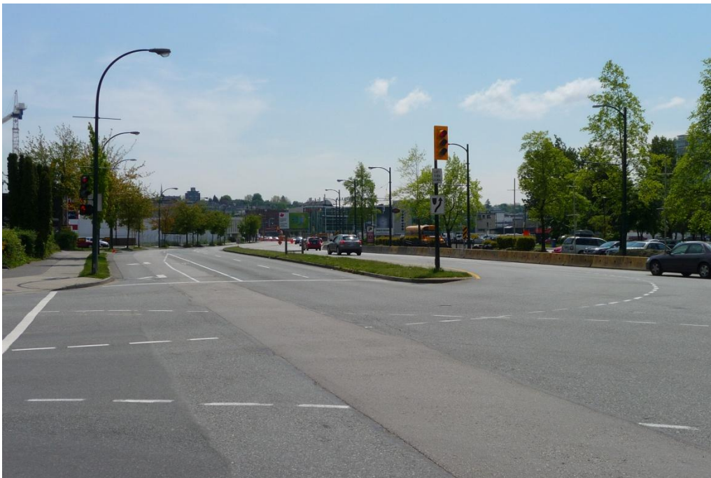
Figure 18 – Intersection of Terminal Ave and Quebec St, facing south, May 31, 2011 (Source: © A. Jones)
