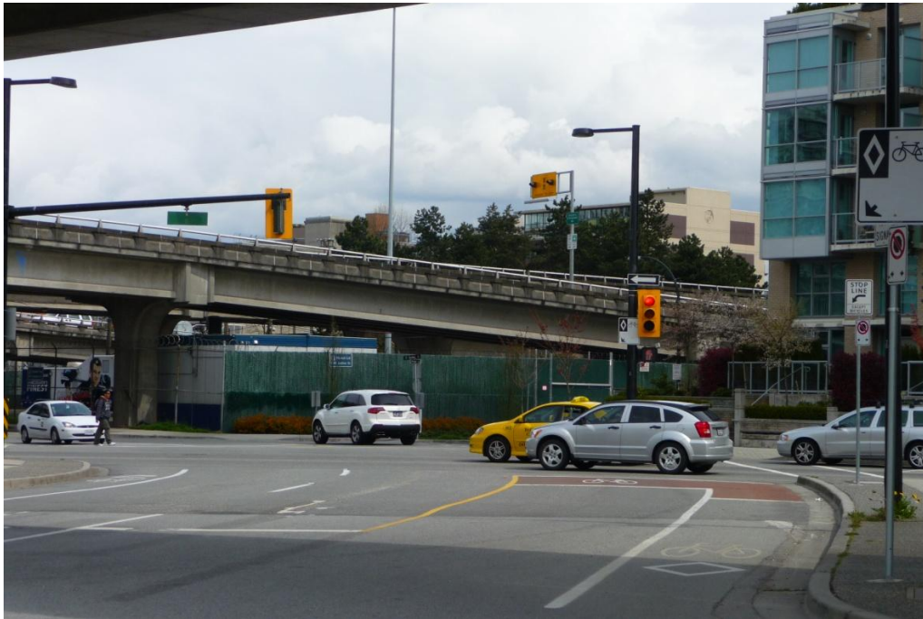
Figure 19 – Viaducts at north end of City Gate on Quebec St, transition zone to Chinatown and BC Place, April 20, 2011 (Source: © A. Jones)
