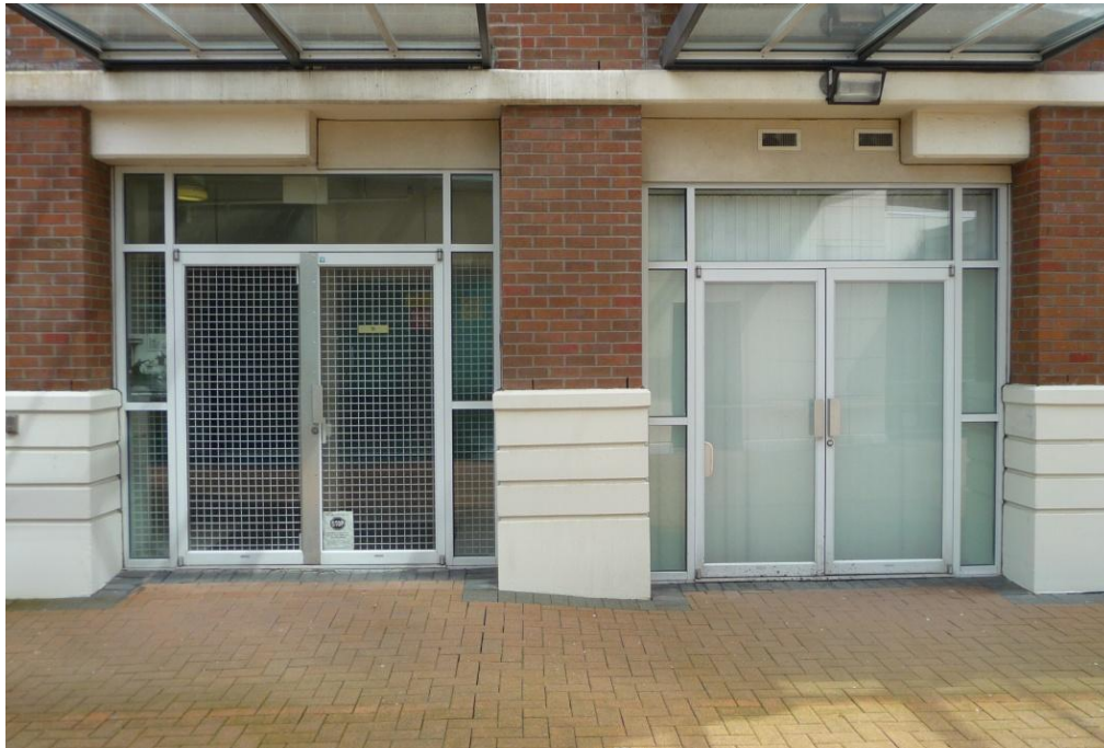
Figure 26 – Unoccupied retail units in City Gate, April 20 2011 (Source: © A. Jones)
