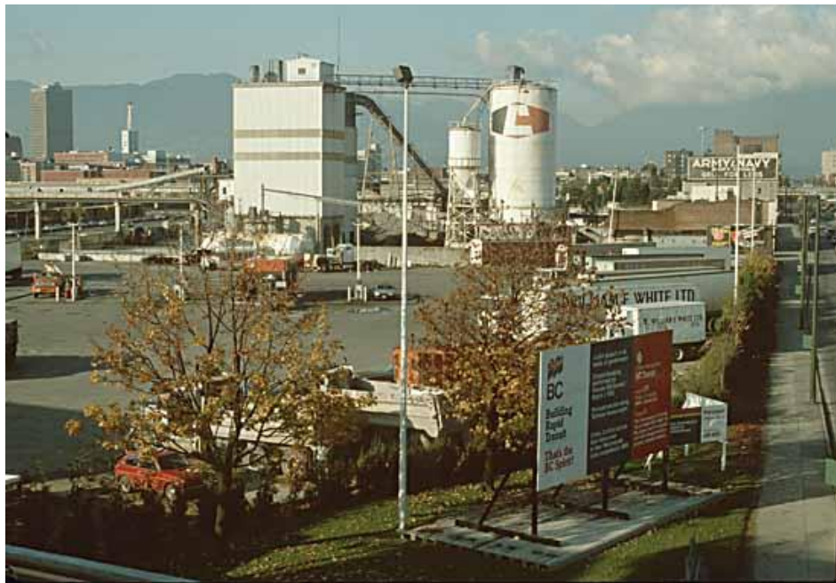
Figure 6 – Main Street Station Site and LaFarge Concrete Plant, Source: © City of Vancouver (City of Vancouver, 1983)
