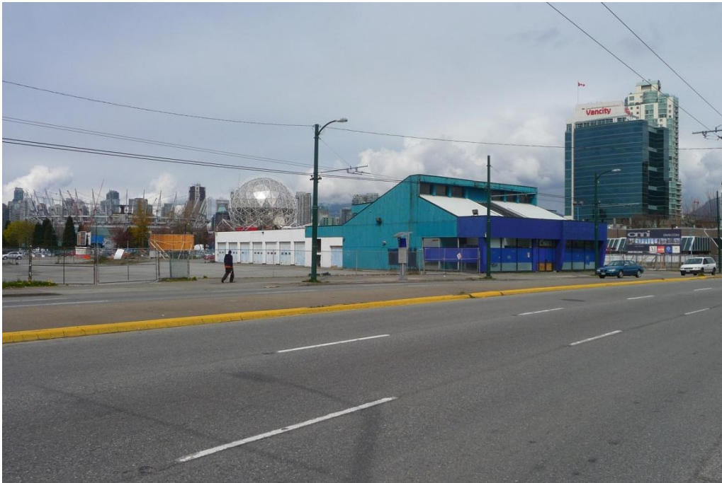
Figure 11 – Vacant land and abandoned building on Main Street south of Station (Source: © A. Jones)
