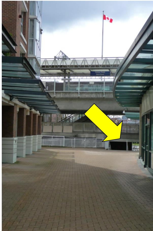
Figure 24 – Access between station and City Gate, north side, April 20 2011 (Source: © A. Jones)
