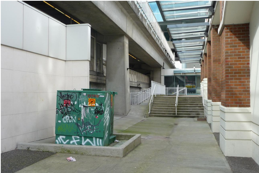
Figure 13 – Impermeable design of station structure as it meets newer buildings on Main Street, east side, April 20 2011 (Source: © A. Jones)
