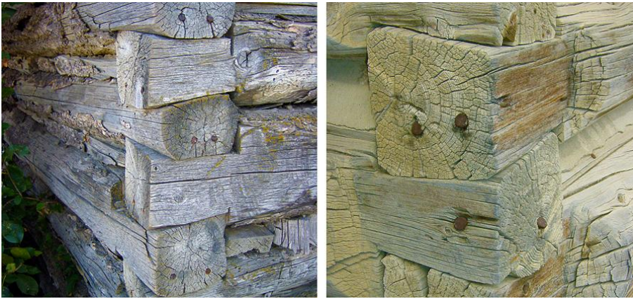
Figure 8. Dovetailed corners on cabins. Left: One-Owl cabin; right: Fort Macleod NWMP detachment. Note the nails on both. Photo by author.
