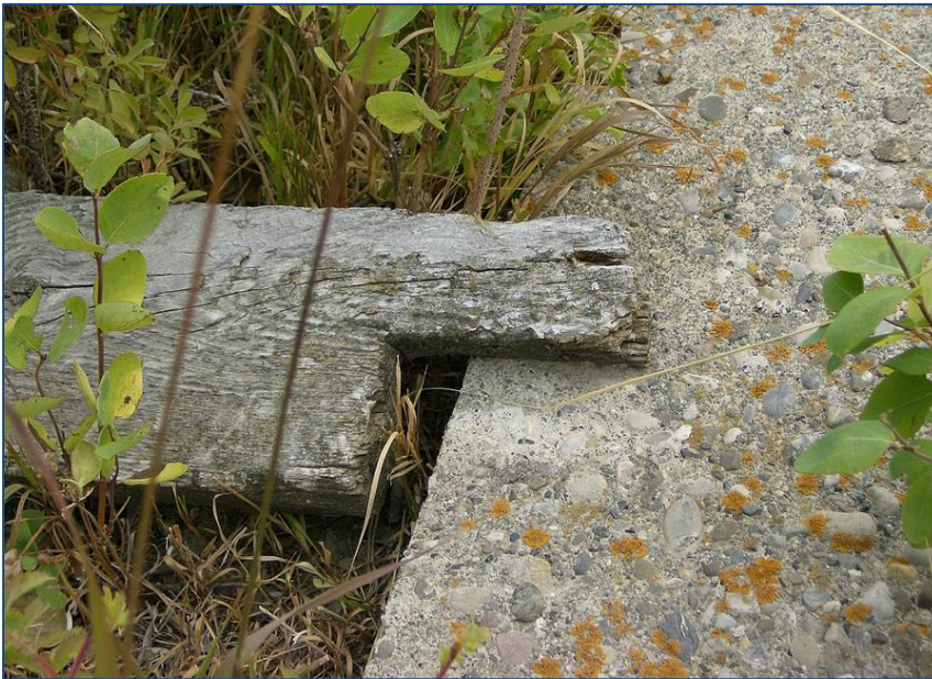
Figure 9. Floor joist from Charlie Grier's cabin on the Piikani Reserve. Not all floor joists were notched to seat the foundation as this one is. Photo by author.
