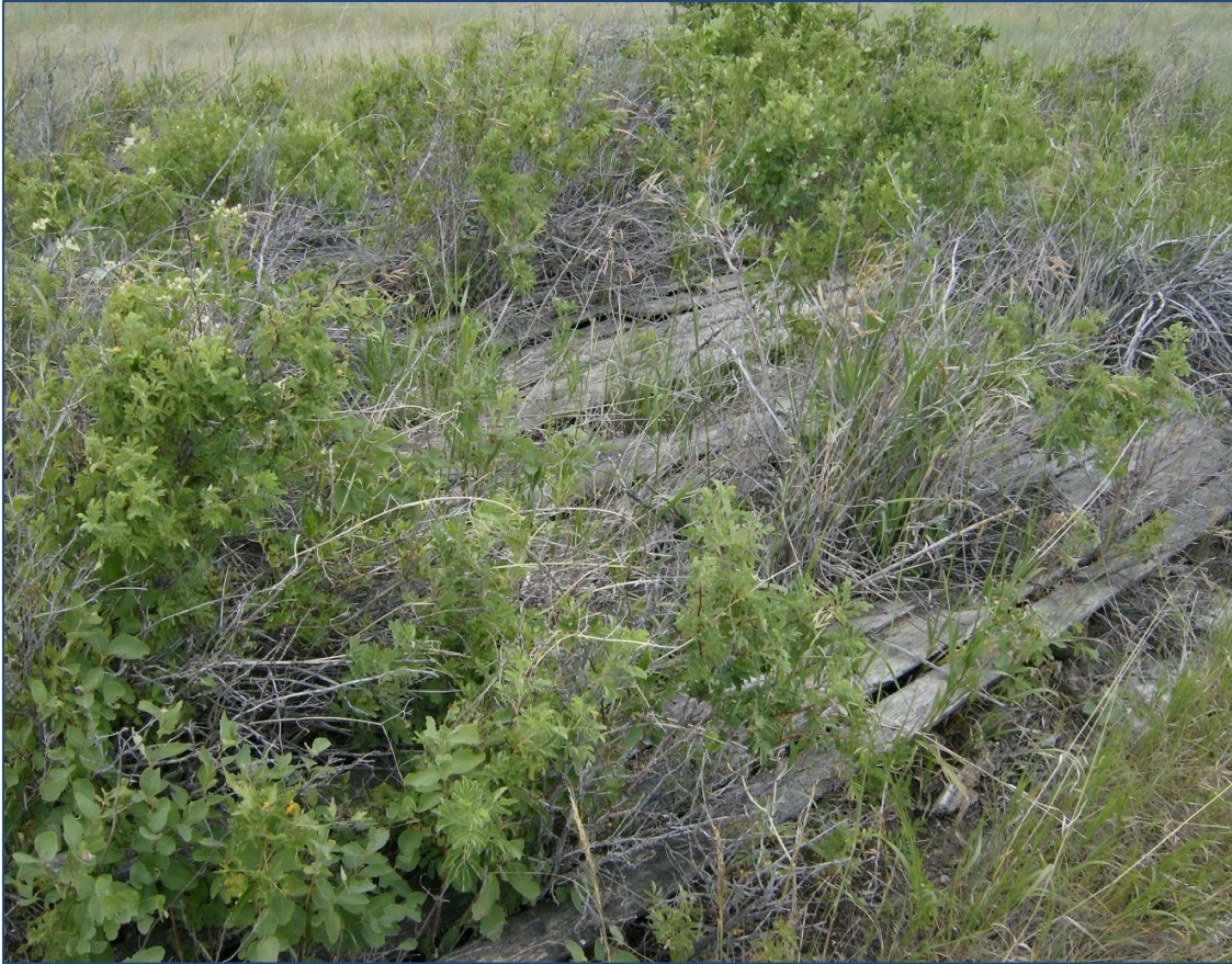
Figure 13. The Yellow Horn cabin foundation, looking north. Photo by author.
