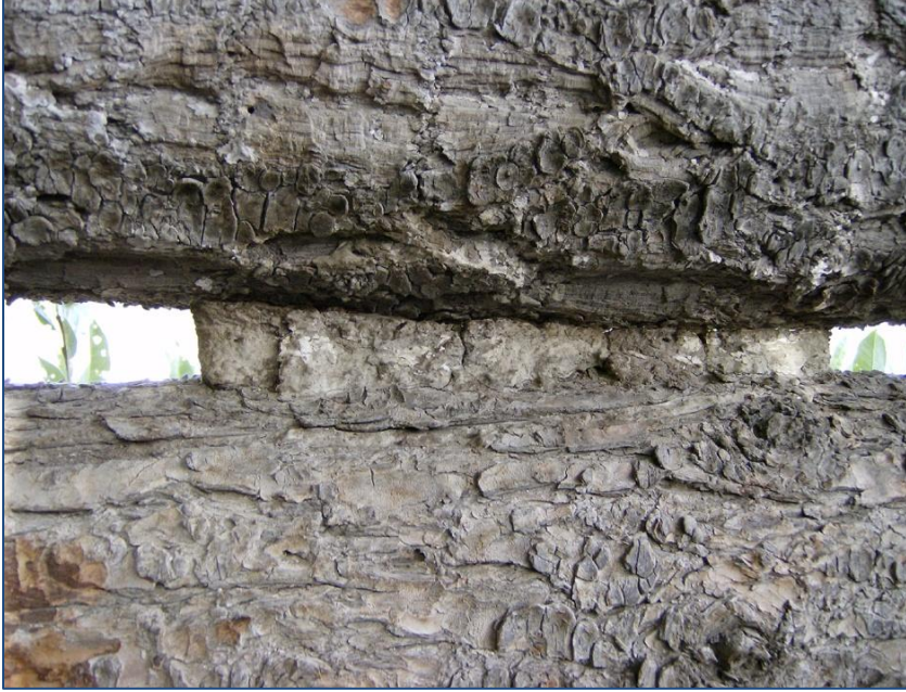
Figure 10. Close-up view of a wall of the One-Owl cabin, looking out. Little remained of the chinking. Photo by author.
