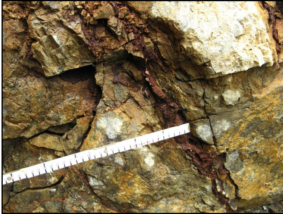
Figure 4.11: Organic layer infilling rock fractures along failure slope. Scale shows 1 cm increments.
