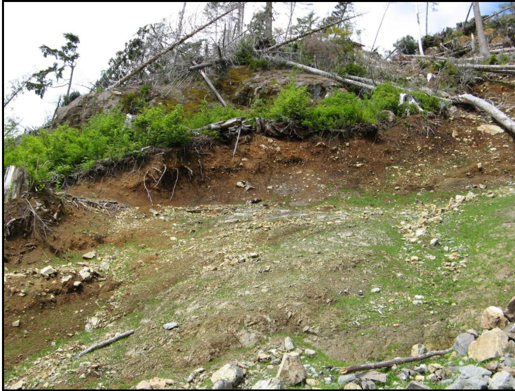
Figure 3.16: Root orientation within face of landslide headscarp. Few vertical tap roots were observed.
