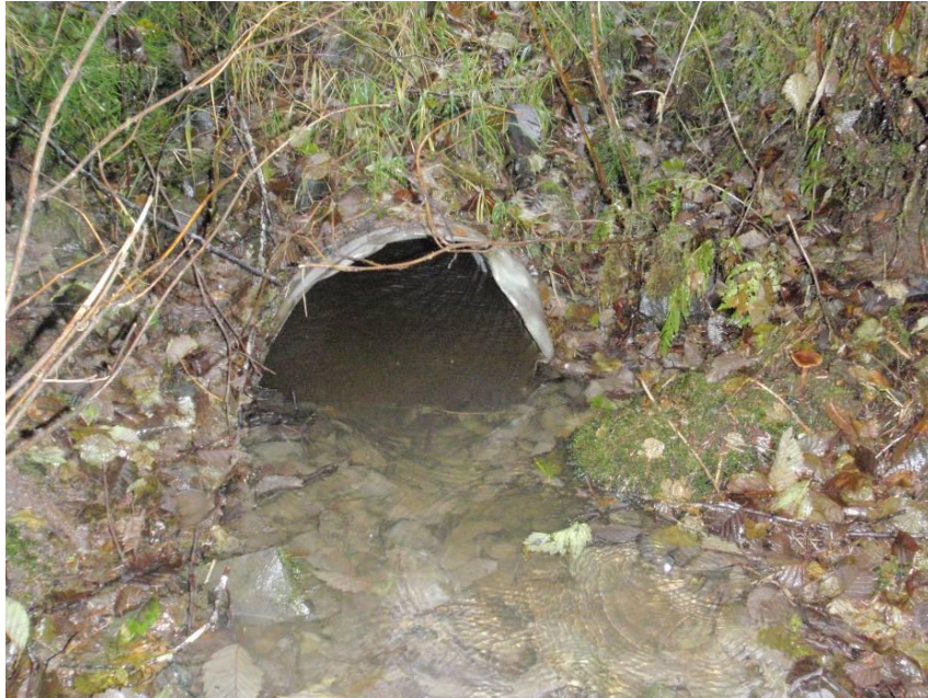
600mm metal culvert at Site 33
