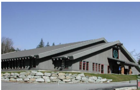
Figure 18 – Squamish Nation – Totem Hall Note: SLCC Archival Materials, photo: Gary Feighen
