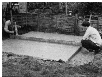
Figure 30 – Laying Concrete
