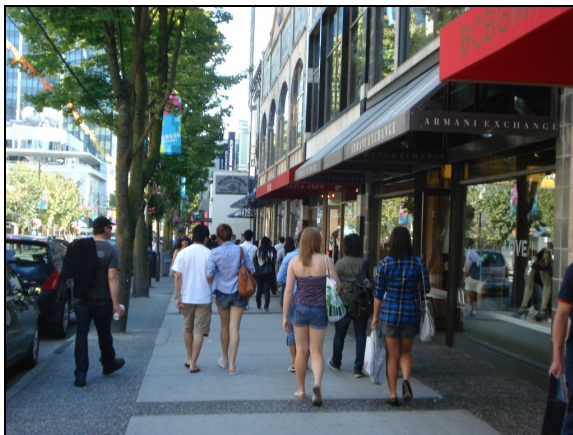
Figure 28: Wider Effective Width and Good Quality Paving and Condition
